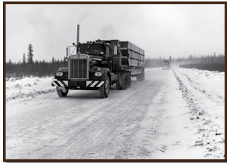
Trucks bound for Bettles and Prospect Creek Camp on ice road during Trans-Alaska Pipeline construction. March 10, 1970.
