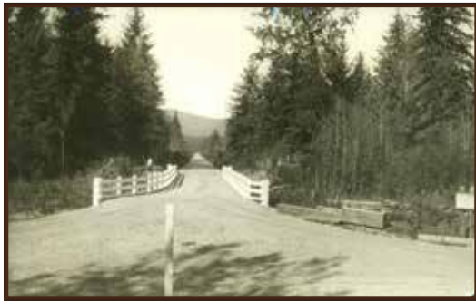
A short bridge along the Glacier Highway near Juneau, built by the Bureau of Public Roads. Alaska State Library, George A. Parks Photo Collection ASL-P240-235
