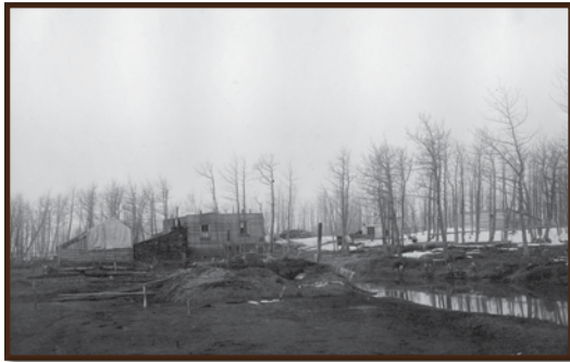
Buildings at Pilgrim Hot Springs, Alaska.
