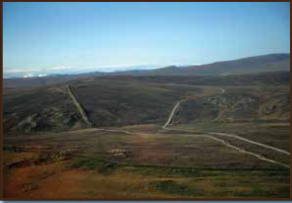
Dalton Highway and Trans-Alaska Pipeline
