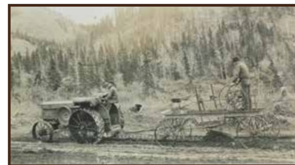
An Alaska Road Commission construction crew grading a road with a case tractor.
