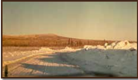
A scene on the Hickel Highway during its construction, April 1969.
