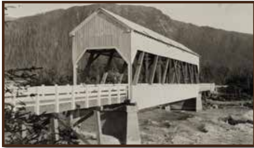
The covered Mendenhall Loop bridge near Juneau. Alaska State Library, U.S. Alaska Road Commission Photo Collection ASL-P61-083-078
