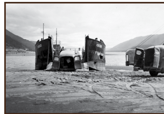
The Haines ferry MV Chilkoot loading a vehicle at Juneau, July 1950. The Chilkoot was a repurposed World War II landing craft that was one of the first ferries in the Southeast.
