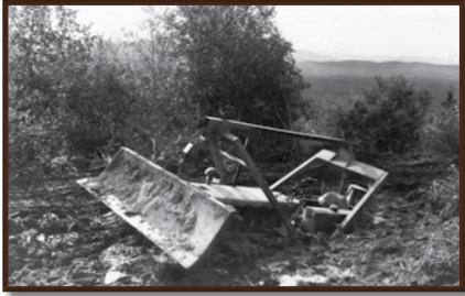
Road construction equipment in deep mud.
