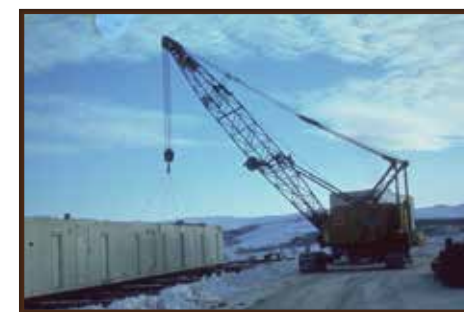
Removing the barracks at the Old Man camp on the Haul Road (now Dalton Highway) during the construction of the Trans-Alaska Pipeline, February 1976. Many of the camps were modular to allow for easy movement along the construction route.
