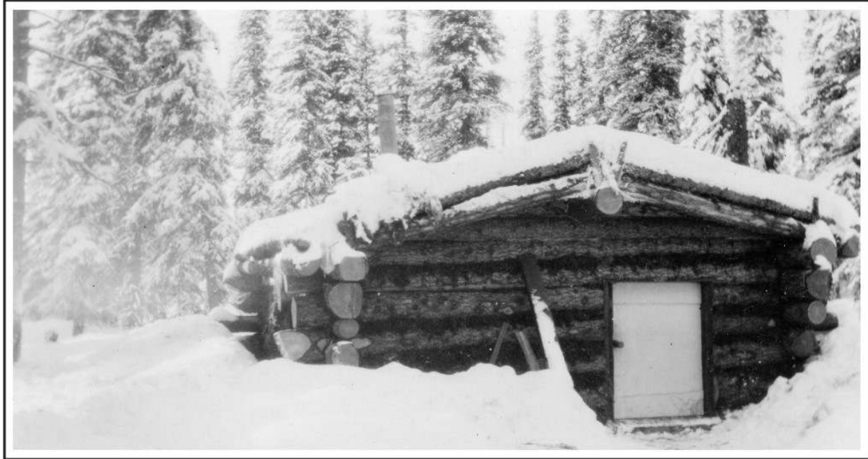
Figure 19. A typical shelter cabin funded by the TBRC and built by the ARC along remote routes such as the Caro-Coldfoot Trail in the 1920s. Photo courtesy of the ADOT&PF Bridge Design Section, Juneau.
