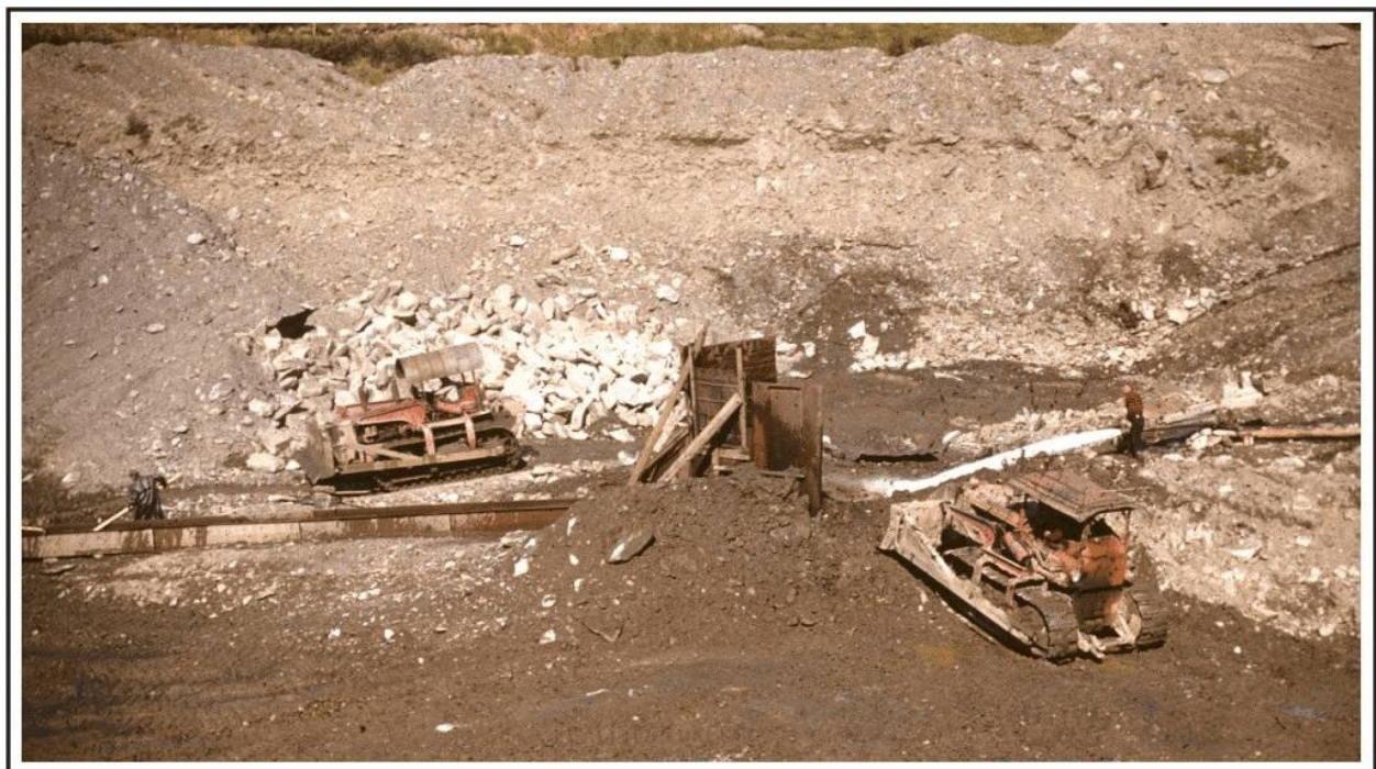
Figure 34. Sluicing using bulldozers at Hugh Matheson’s mine on Big Creek, late 1950s. Slide courtesy of Hugh Matheson, Boulder, Colorado.
