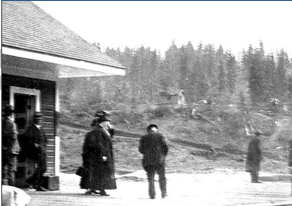
Figure 9: Photo courtesy of Judy Block. Origin is unknown. Railroad depot at left was constructed after the Chitina Cemetery Road was constructed according to other photography. A photo dated March 1, 1912 has depot and road, but not bunkhouse. Note: residence on hill
