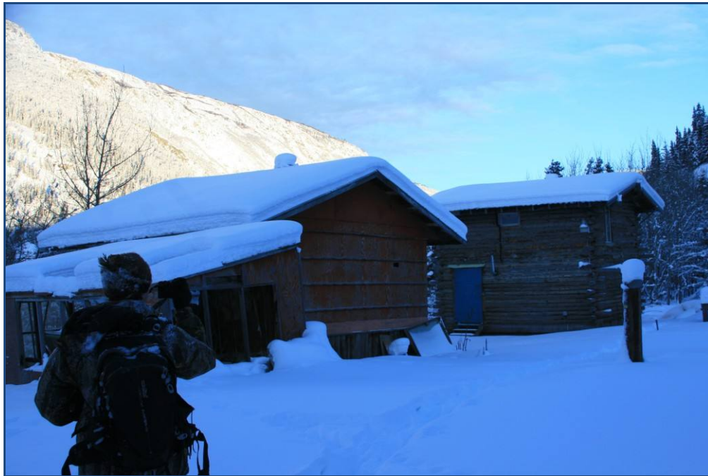
Figure 16: Photograph by Kevin Sorensen, DNR PAAD Unit, January 21, 2010. Jason Cheney, ADF&G in foreground. Photo of the residential structures on Ammi property, Lots 8-10, Block 6.
