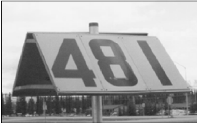
Figure 31. Pipeline marker for aerial surveillance. From collection of USARAK.
