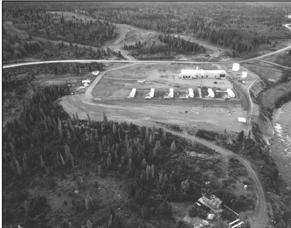
Figure 33. Blanchard River Pump Station. NARA.
