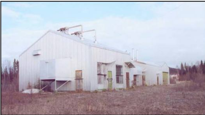
Figure 41. Timber Pump Station, May 2002. From collection of USARAK.
