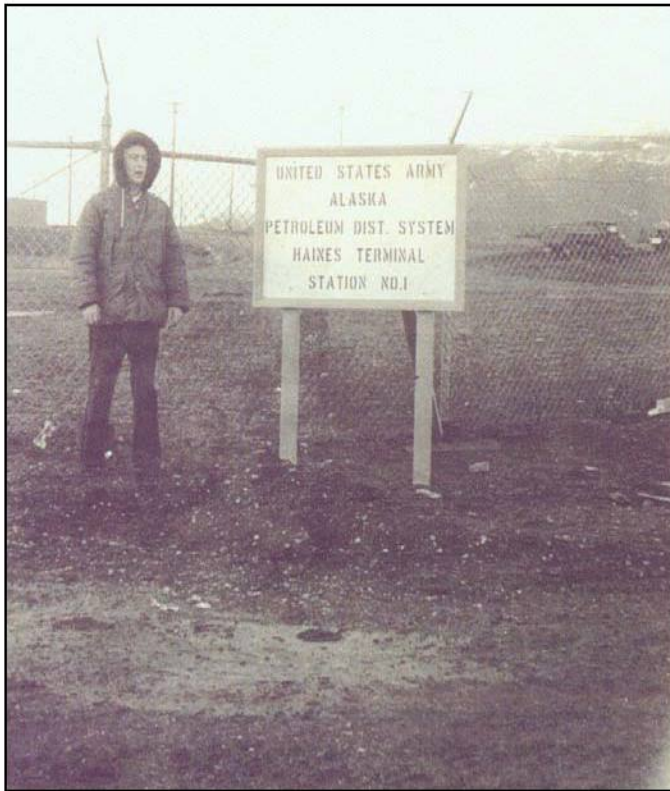
Figure 36. Byrd Kelley at the Haines Terminal front gate, ca. 1957. Courtesy Jeannette Menaker.
