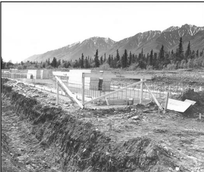
Figure 32. Destruction Bay under construction. NARA.
