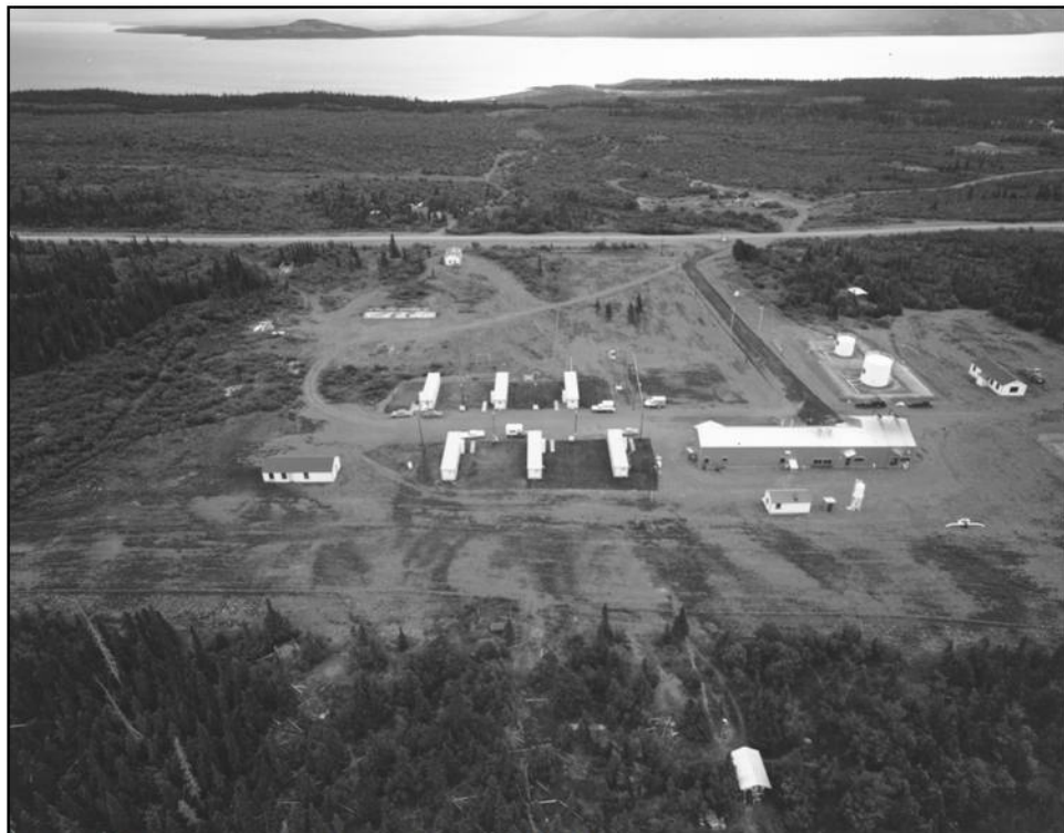
Figure 34. Destruction Bay Pump Station. NARA.
