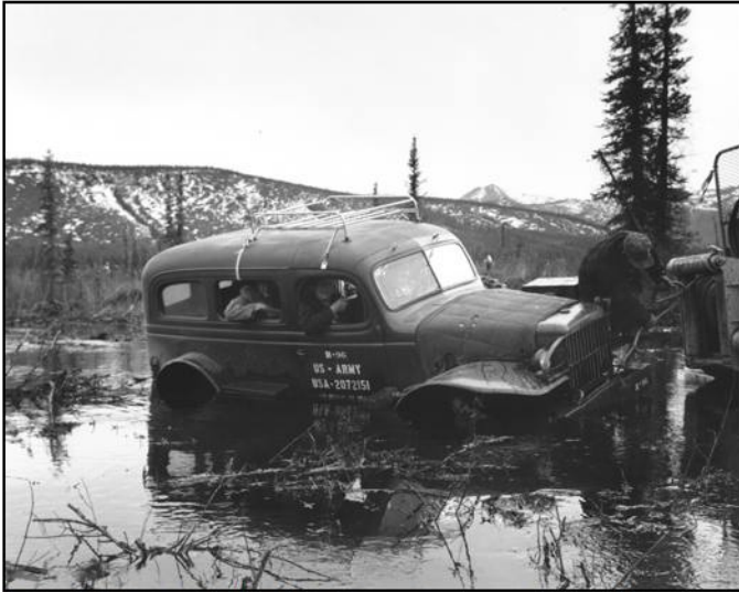
Figure 8. Area 2. Mile 1173, Yukon Territory, Corps of Engineers inspection vehicle mired along pipeline right-of-way. NARA.
