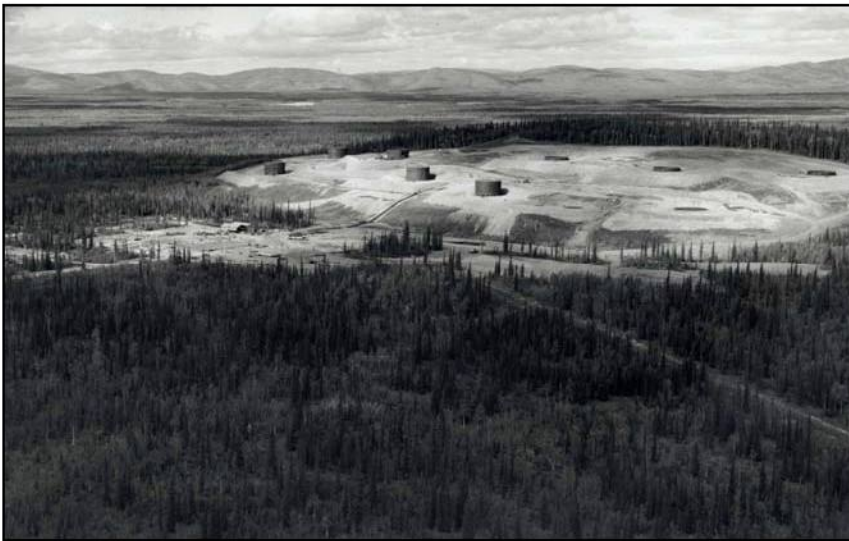
Figure 9. Tok terminal under construction, 1954. NARA.
