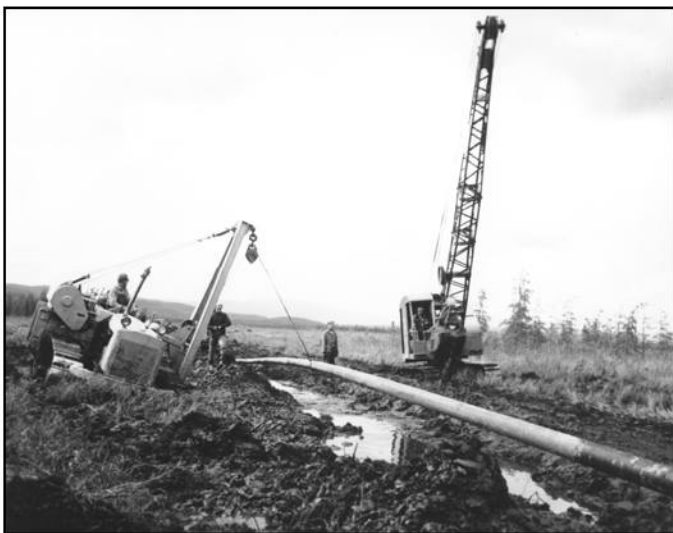
Figure 6. Pipeline construction. NARA.
