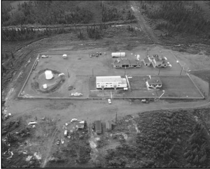
Figure 18. Donjek Pump Station. NARA.
