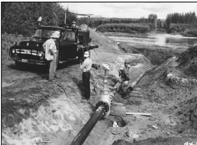
Figure 5. Laying pipe for underwater crossing. NARA, A4-3826.
