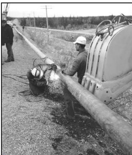
Figure 7. Pipe welding. NARA, DA 573 #373.
