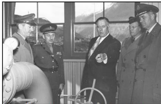
Figure 13. Tom Nelson, superintendent of the Haines-Fairbanks $40,000,000 POL pipeline, explains to distinguished military guests how the great ALCANGO 626-mile pipeline carries the different fuels, jet and aviation, motor and diesel, to military bases in the interior. L to R; Maj. Gen. James F. Collins, Commanding General USARAL; Brigadier H. L. Meuser, Commander, Northwest Highway System, Canada; Brig. Gen. Hugh Mackintosh, Columbus General Depot, Quartermaster Corps; Lt. Gen. J. H. Atkinson, USAF Commander in Chief, Alaska; Commissioner, F. H. Collins, Yukon Territory, Canada. U.S. Army photograph, Sheldon Museum Collection, Haines, Alaska.
