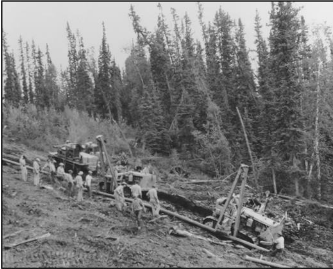
Figure 11. Haines-Fairbanks Pipeline construction. NARA.
