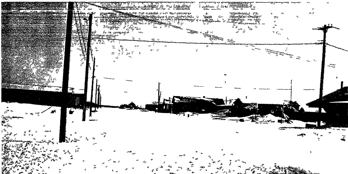
Main Street at Emmonak. Note utility poles and lines.
