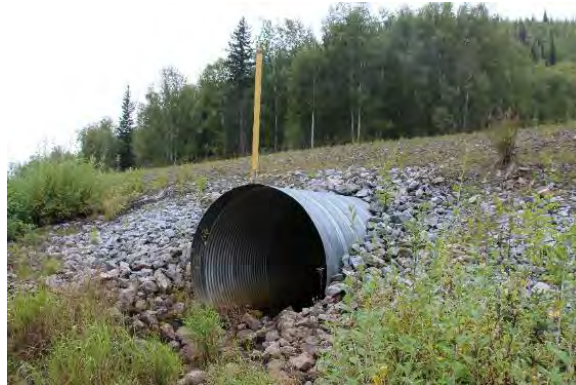
Figures 45 (view facing west) and 46 (view facing southwest). Replacement culverts (one with thaw pipe).
