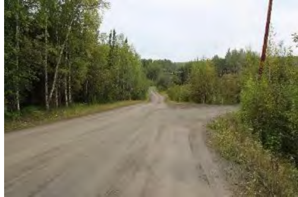
Figure 56. Single-lane gravel roadbed transition into widened portion of section near eastern terminus/intersection with Segment B of the Elliott Highway. View facing west.
