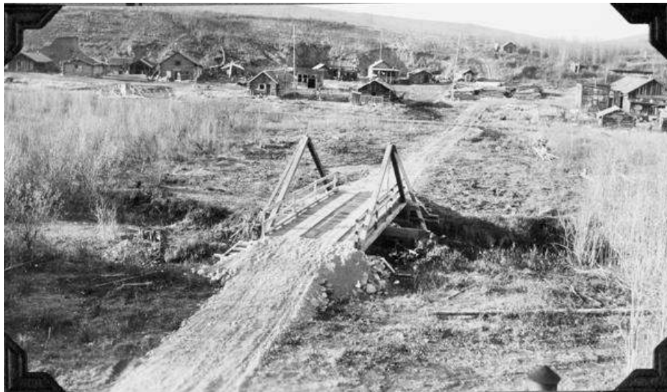
Bridge crossing Livengood Creek in Livengood, c.1938.
