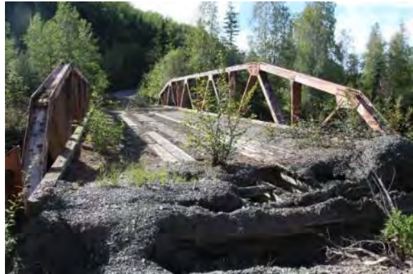
Figure 32. 1949 Warren pony truss bridge reflective of pre-1959 period of significance (does not connect to gravel roadbed) – over the Tatalina River. View facing south.
