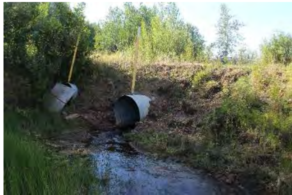
Figures 17 (view facing northeast) and 18 (view facing south). Typical replacement corrugated metal culverts (one with thaw pipe).
