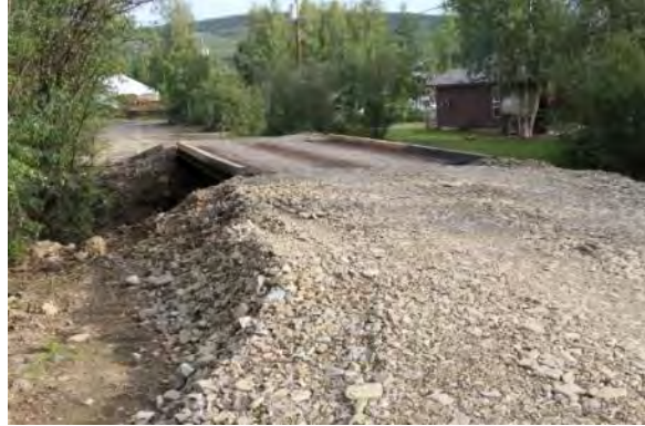
Figure 21. Replacement bridge. View facing north.
