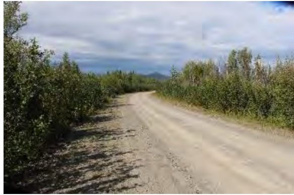
Figures 49 (view facing southeast) and 50 (view facing north). Gravel roadbed with embankment and two travel lanes reflective of pre-1959 period of significance.
