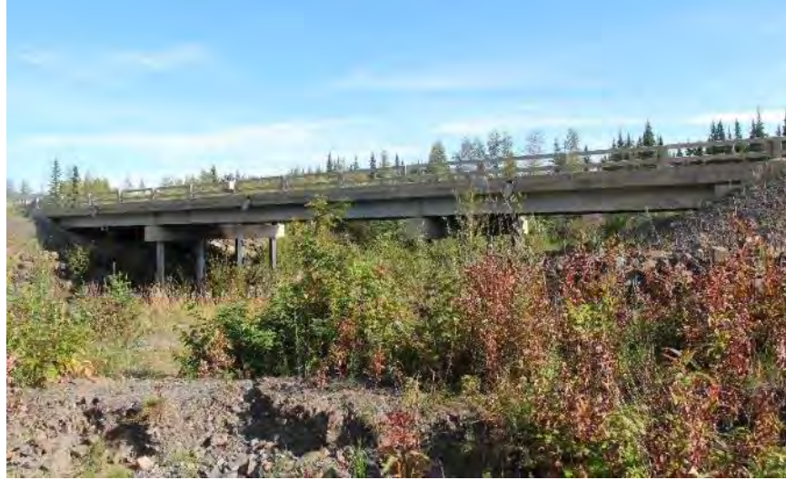
Figure 16. Example of a replacement bridge. View facing north.
