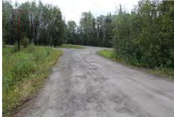
Figure 57. Gravel roadbed with two travel lanes and embankment eastern terminus/intersection with Segment B of the Elliott Highway. View facing east.
