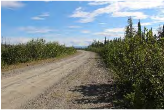
Figures 49 (view facing southeast) and 50 (view facing north). Gravel roadbed with embankment and two travel lanes reflective of pre-1959 period of significance.
