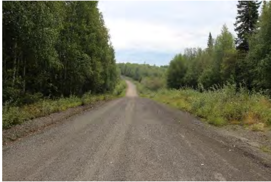
Figure 42. Gravel roadbed east of Manley Hot Springs. View facing northeast.
