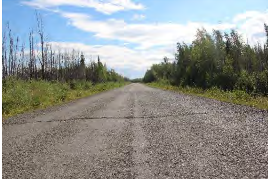
Figure 43. Paved roadbed east of Manley Hot Springs. View facing southwest.
