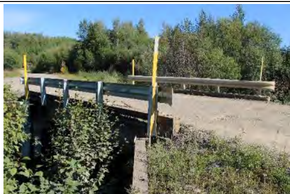
Figure 36. Replacement bridge in Livengood. View facing north.
