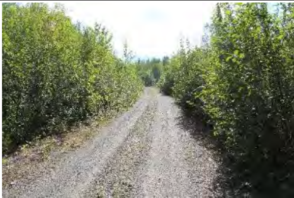
Figure 51. Gravel roadbed with single travel lane reflective of pre-1959 period of significance. View facing south.
