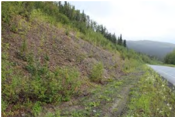
Figure 8. Roadside cut. View facing northeast.
