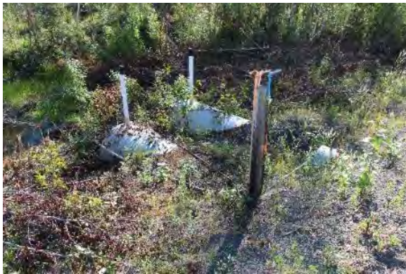
Figures 17 (view facing northeast) and 18 (view facing south). Typical replacement corrugated metal culverts (one with thaw pipe).
