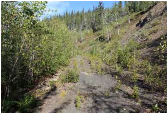
Figure 27. Example loss of travel lanes (unmaintained). View facing northwest.
