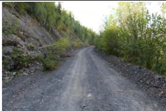
Figure 30. Gravel roadbed, one travel lane, and embankment reflective of pre-1959 period of significance – south of the Tatalina River. View facing south.
