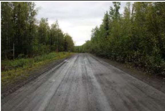
Figure 29. Gravel roadbed, two travel lanes, and embankment reflective of pre-1959 period of significance – south of the Tatalina River. View facing east.
