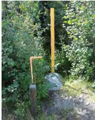
Figures 45 (view facing west) and 46 (view facing southwest). Replacement culverts (one with thaw pipe).
