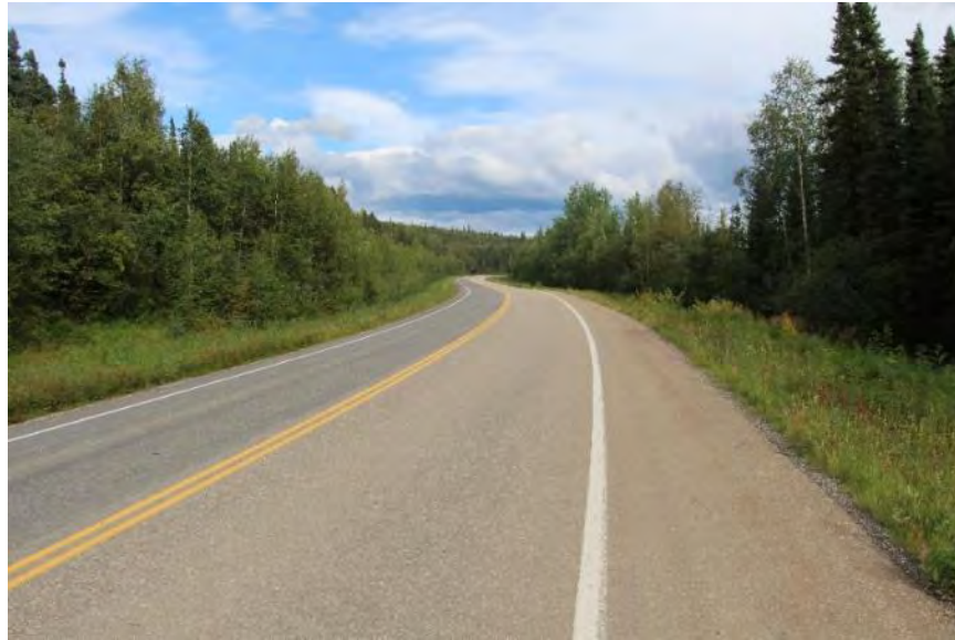
Figure 5. Typical roadbed showing wide shoulder. View facing east.
