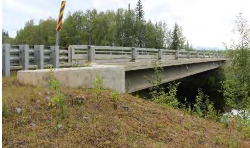
Figure 44. Replacement bridge. View facing south.
