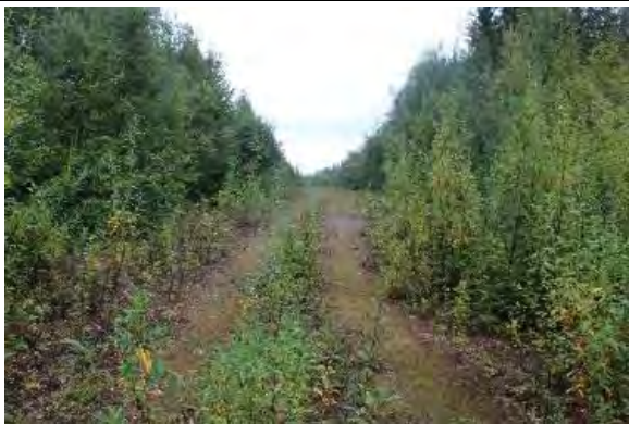
Figure 53. Example loss of embankment and travel lanes. View facing north.
