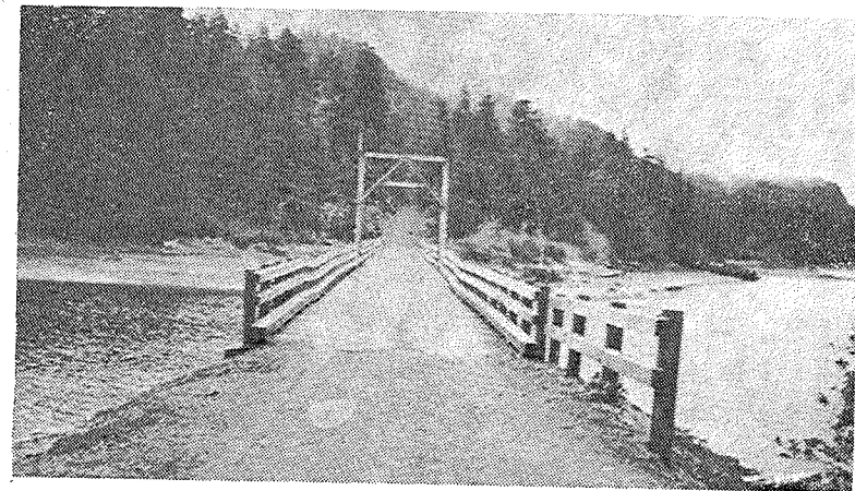
KLAWAK BRIDGE BEFORE REPAIRS
