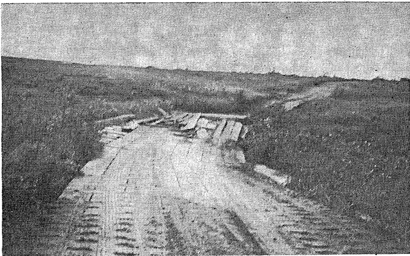
SOUTH NAKNEK ROAD BEFORE REPAIRS
