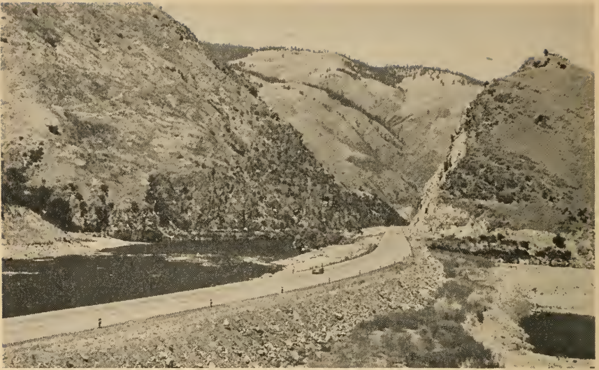
This Federal-aid project on U.S. 95 along the Salmon River near Freedom, Idaho, required a 1,500-foot relocation of the river channel and a rock cut 400 feet deep.
