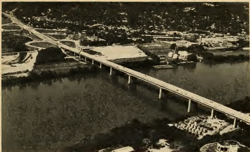
The Olgiate Bridge over the Tennessee River at Chattanooga, Tenn., built with Federal-aid funds, links a series of improvements on Interstate Route 124 and U.S. 27. The old Market Street Bridge nearby was a focus of frequent traffic jams.
