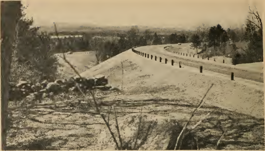
On Interstate Route 89 in Hopkinton, N.H., independent roadway design provides a high degree of safety and eliminates headlight glare at night. One roadway lies atop a ridge while the other is downhill and across a scale.
