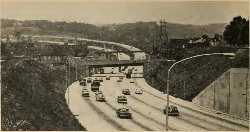
The Roosevelt Expressway in Philadelphia, Pa., was completed with Federal aid during the year. This controlled-access route will relieve overcrowded U.S. 1 and cut travel time in the area it serves. In the background are twin 2,000-foot-long high-level bridges over the Schuylkill River.
