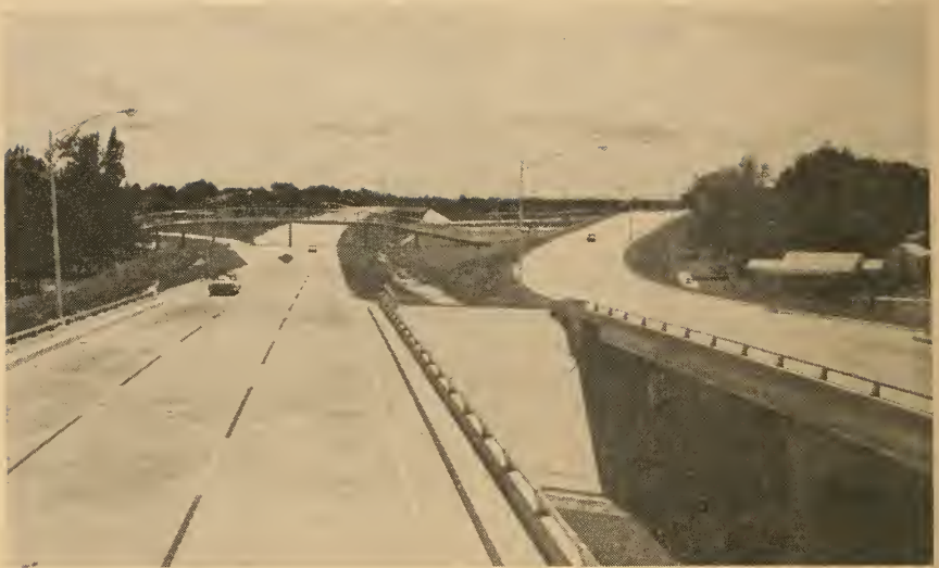
This project on Interstate Route 4 in Orlando, Fla., included a pedestrian overpass providing access to a school.
