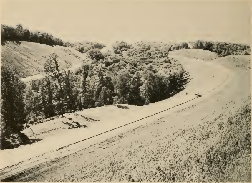
This section of Interstate Route 94 in Wisconsin was designed as two separate roadways, for safety, economy, and pleasing appearance (photograph taken prior to opening to traffic).
