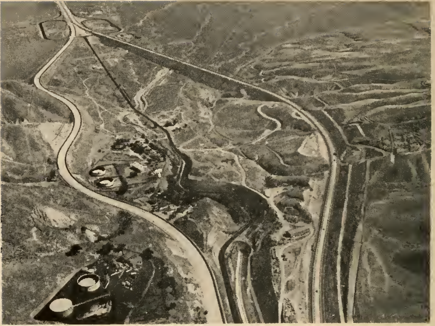
Interstate Route 5, an eight-lane highway south of Bakersfield, Calif. The old four-lane road was improved and used as one of the twin roadways.
