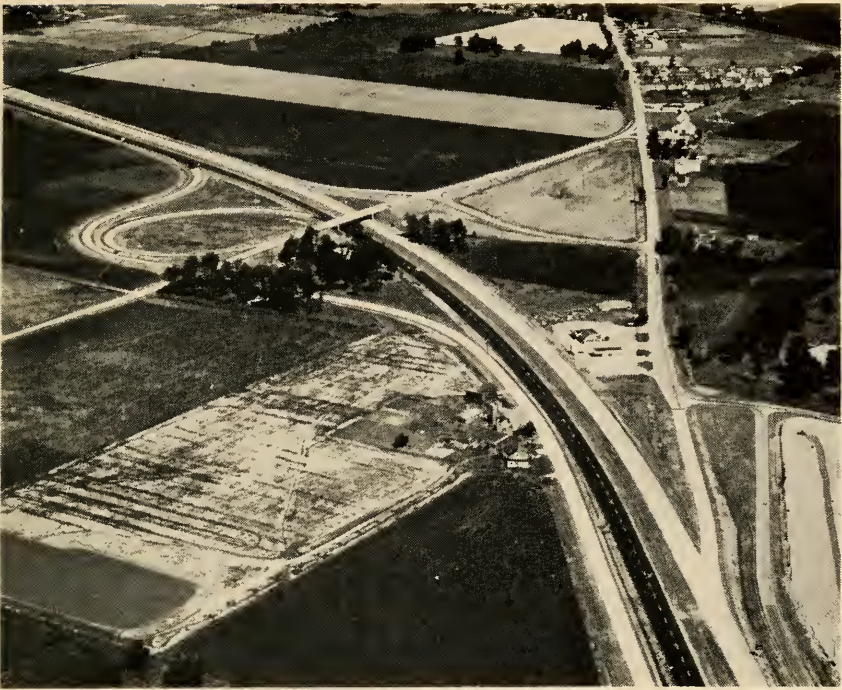
Interstate Route 65 bypassing Lebanon, Ind. Access control was acquired along the existing two-lane bypass and it was used as one roadway of the divided freeway.
