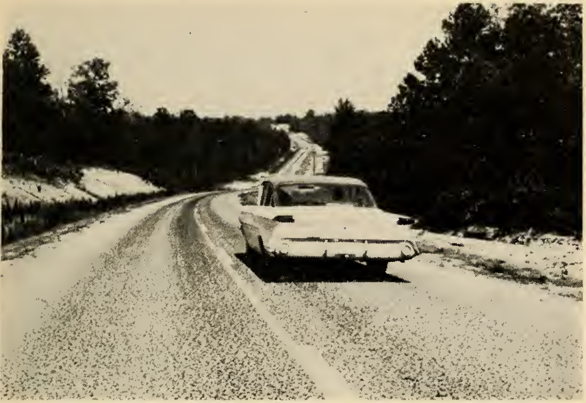
Federal-aid secondary and "D" funds were used to improve 6½ miles of Mississippi Route 18 in Clarke County. Grading, drainage, and a 20-foot bituminous pavement were completed at a cost of $54,000 per mile.
