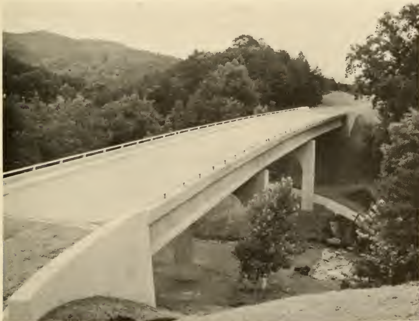
A prestressed concrete bridge carrying the Blue Ridge Parkway south of Roanoke, Va.
