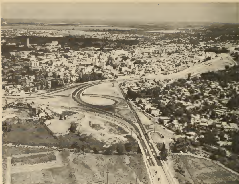
Federal-aid assumes sizable proportions in the Caribbean as shown in this view of a recently completed primary project in Rio Piedras, south of San Juan, P.R.
