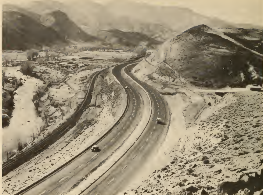
Separate roadway design enhances the vista and reduces the effects of headlight glare on this scenic section of Interstate Route 80 through the Truckee River canyon in Nevada. (Full control of access will be ultimately acquired.)
