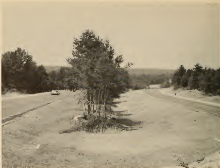
Interstate Route 89, west of Concord, N.H., showing the wide median and independent roadway design, preserving the natural growth in the median.
