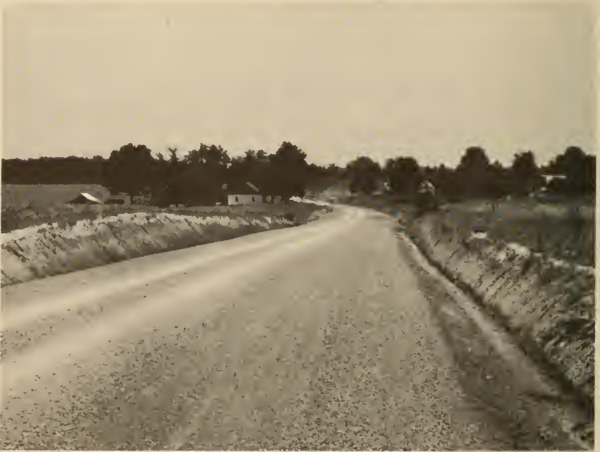
A well-graded gravel road, built with secondary funds, serves the farming and livestock producing communities in Coffee County in south-central Tennessee.
