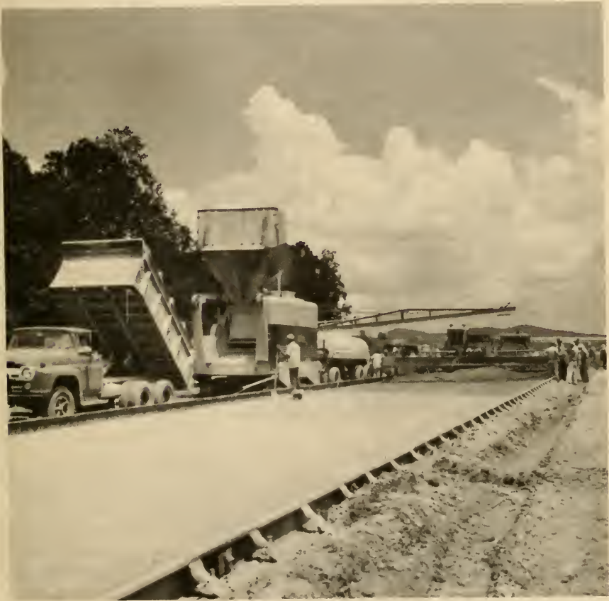
Paving operations on Interstate Route 40 in North Carolina
