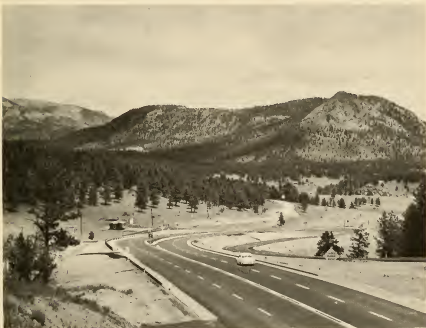
A recent primary project, near Bailey, Colo., removed a number of treacherous curves and steep grades on U.S. Route 285 through the Colorado Rockies. The basic two-lane section in this area was widened where necessary to provide for truck lanes and channelization of intersections.
