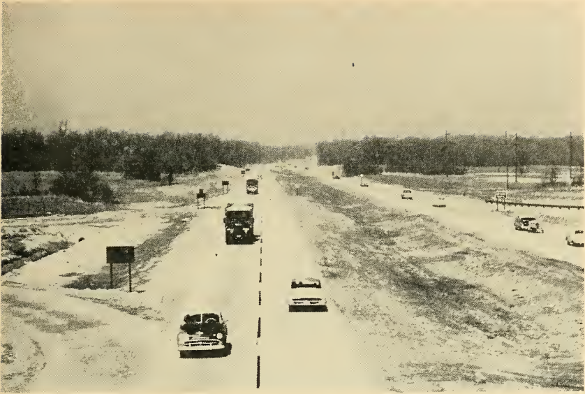
The 23-mile Farmington-Brighton Expressway, part of the Interstate route from Detroit to Muskegon, Mich., was completed during the year.
