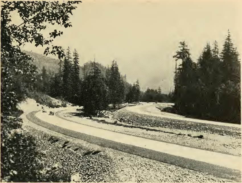
This Washington State Interstate route follows the historic path of pioneers through Snoqualmie Pass in the forested Cascade Range, 40 miles east of Seattle.
