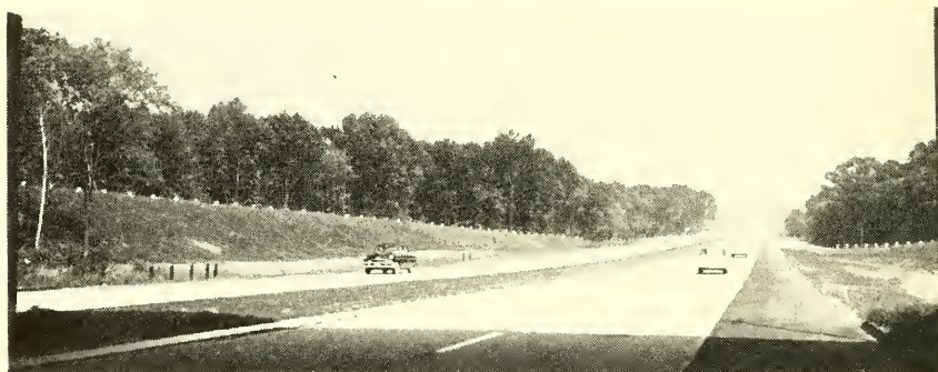
The Windsor section of the Hartford-Springfield Expressway, a relocation of U. S. 5 in Connecticut.
