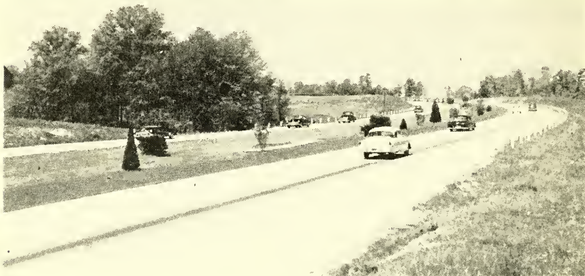
A section of the Interstate System about 15 miles west of Baltimore, Md., that coincides with U. S. 40. Center planting will prevent headlight glare. This completed highway does not meet the new standards in all respects, for while important cross roads have grade separations some county roads cross at grade and there are a few private entrances. No commercial establishments have direct access.
