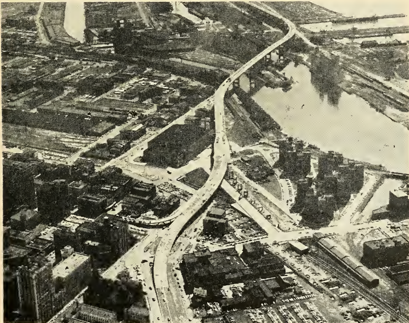
The Buffalo (N. Y.) Skyway, a 49-span structure passing over a river, a canal, two railroads, the Niagara Thruway, and a number of city streets, carries about 18,000 vehicles a day and relieves congestion in the main business district.
