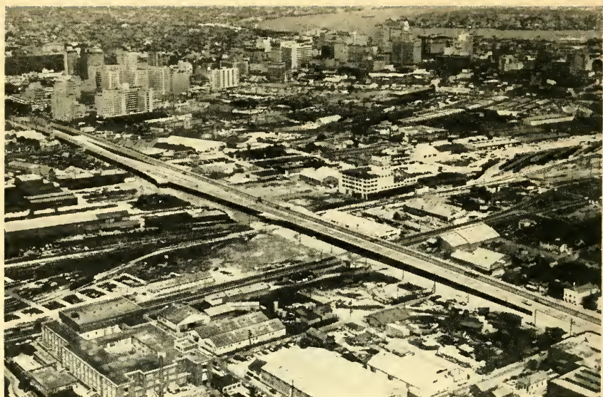
Elevated 6-lane expressway in New Orleans.
