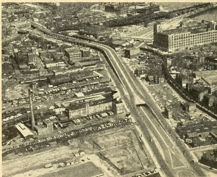
The new three-level Sullivan Square Expressway in Boston.
