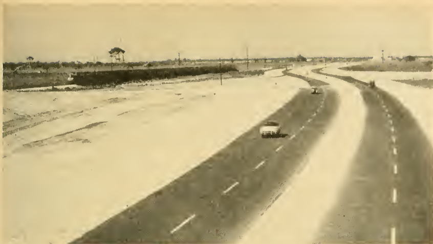
Wide right-of-way and control of access are important features of this improvement on the interstate system near Miami, Fla.
