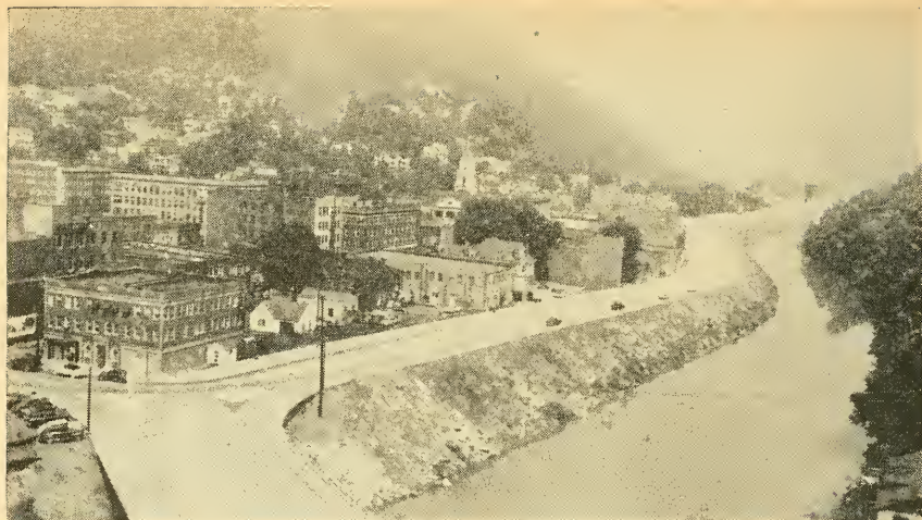
Relocation of U. S. 119 through Logan, W. Va., in a narrow valley where all space was occupied, was accomplished by building the new highway on a rock fill in the river.
