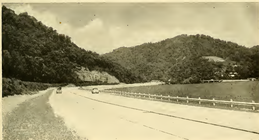
The four-lane divided highway completed at Gauley Bridge in West Virginia.
