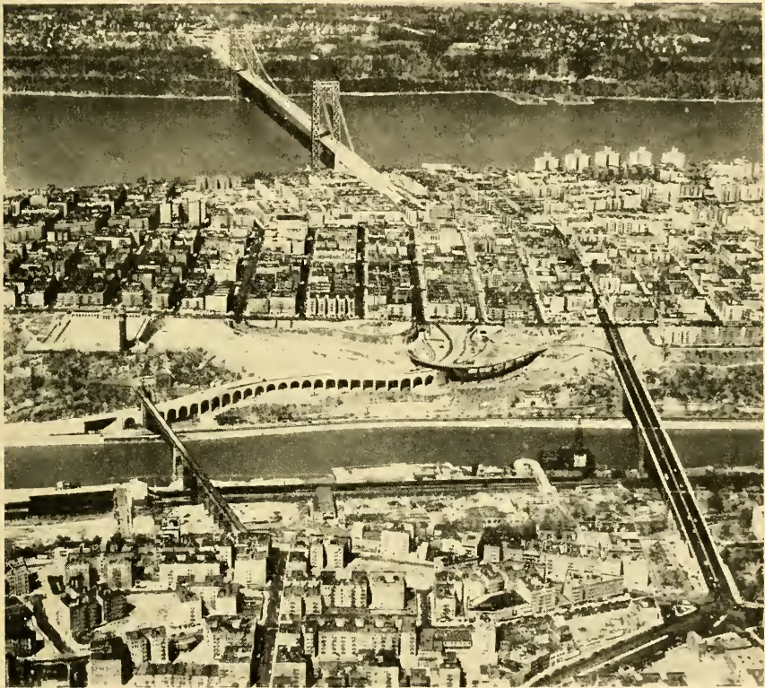
The Highbridge Interchange in New York City
