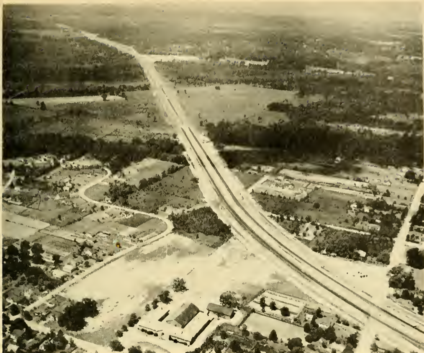
The new four-lane highway on U S 90 approaching Mobile.
