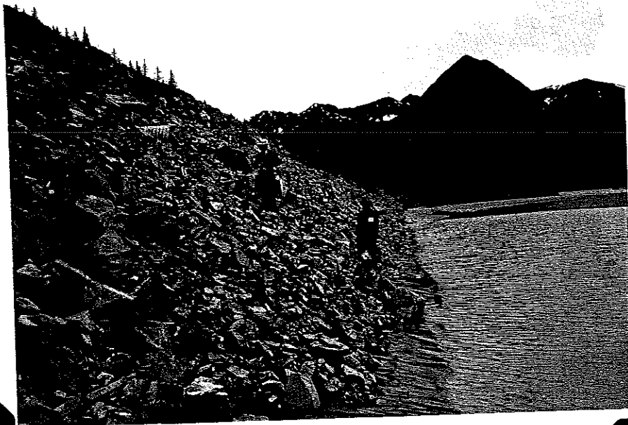
Turnagain Arm, F-2. View of roadway fill along Turnagain Arm tide flats about two miles south of Girdwood. The culvert pipe outlet shown in the picture was at the elevation of the silt when the culvert was installed. The silt was eroded away by tidal currents leaving the outlet about 12 ft. above the present elevation of the silt below. (#1703)
