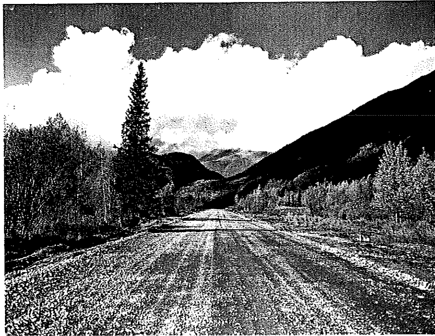
Seward-Anchorage Highway, Sec. B-2. View north from about Mile 37 \frac{1}{2} . Shows new grading with borrow course in place. (#1924)
