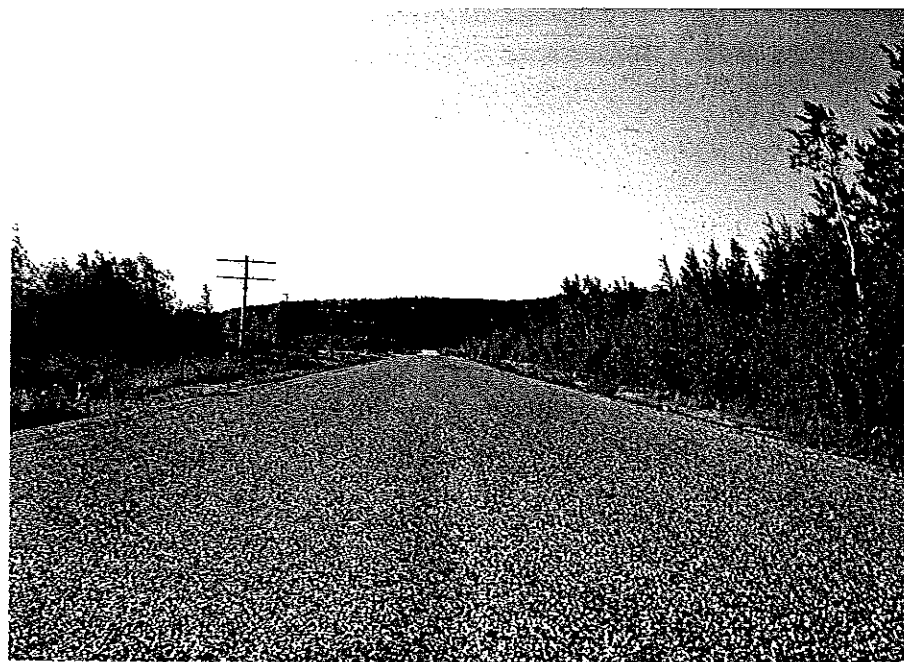
1416. DMF-40-4. Richardson Highway, Sec. A. View south from 41 miles south of Fairbanks. Shows cover aggregate on finished surface one year after completion of paving.
