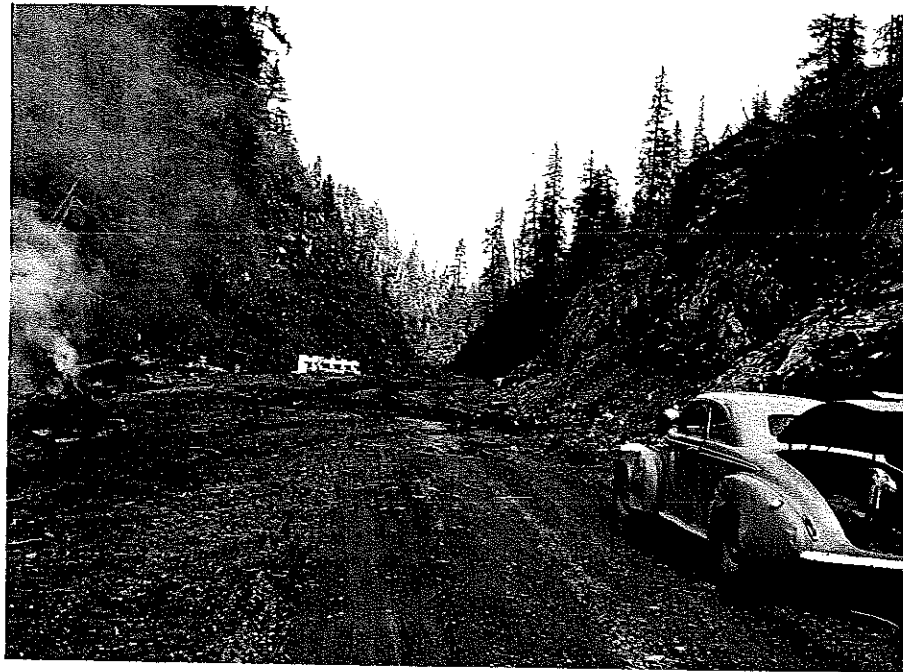
1465. DMF-43-5. Seward-Anchorage, A-1. View of a narrow section of Grouse Canyon. Shows old bridge at Sta. 1449. New centerline goes through the hand-rail on the right side of bridge. The large cut to be made on the left, ahead of the bridge, is for a channel change. The bridge is eliminated and new road remains right of the Creek.
