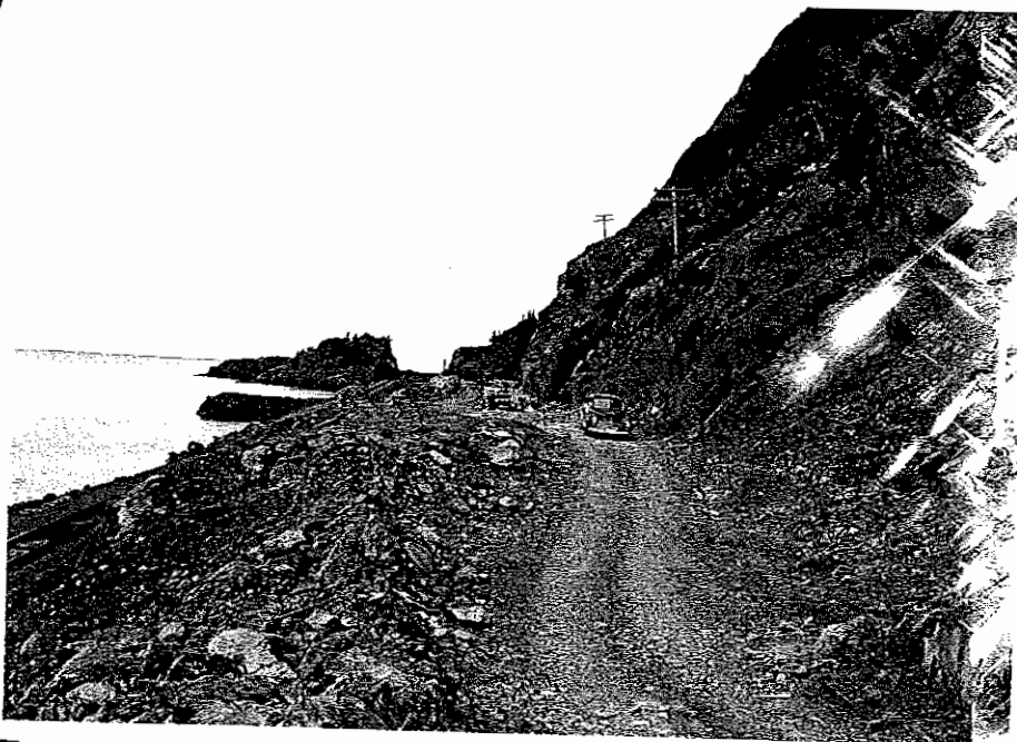
1469. DMF-c.f.41. Turnagain Ave, Sec. 6. View of old Alaska Railroad grade under construction for new highway. New railroad grade is on the left.
