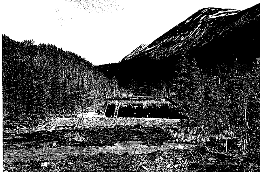
1468. DMF-43-8. Kenai River Highway, 5-B2. View of 150" sectional plate pipe partially assembled. Pipe is to be installed in Daves Creek.
