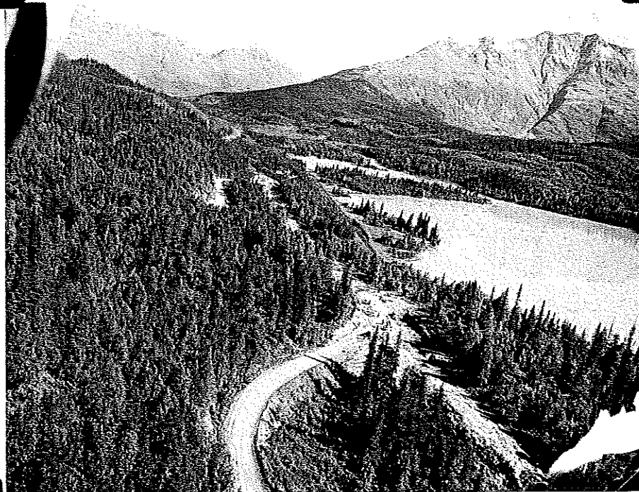
Seward-Anchorage A2, B3. Aerial view north from over about mile 26. Shows curves in old road and clearing for new road. The Alaska Railroad and Lower Trail Lake are right of the new road. (#1761)
