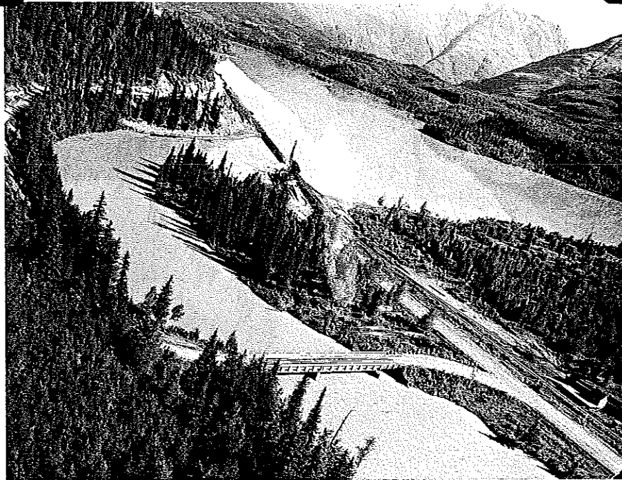
Seward-Anchorage, A2, B3. Trail River at outlet of Lower Trail Lake at Mile 26. Old road crosses on bridge in foreground and goes through 518 degrees of curvature in getting beyond the new bridge site within the limits of this picture. The new road is parallel to railroad and goes through only 15 degrees of curvature within the limits of the picture. The pile driver is working on the new highway bridge. (#1757)
