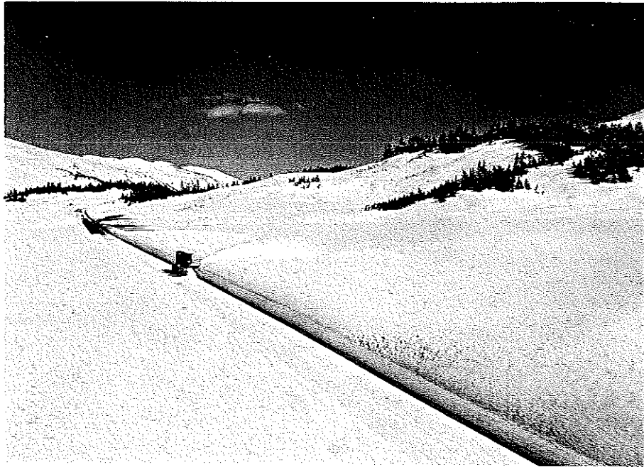
BMF 30-4. #1234. Turnagain Arm D. Aerial view of rotary plow, Snago, on the Granite Creek side of the summit south of Turnagain Arm. Snow at this point is about 7 ft. deep on the level. Maximum depth this year on the summit about a mile behind the plow was 9\frac{1}{2} ft.
