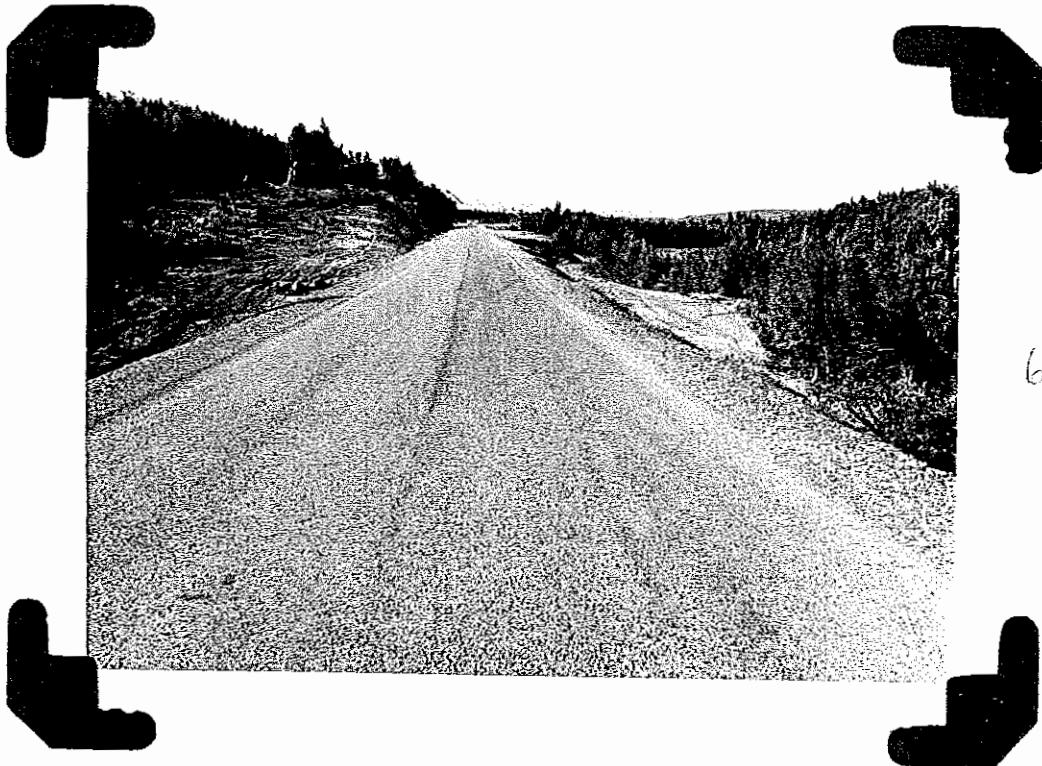
EHC-851 Glenn Highway Sec. A. View of completed paving after seal coat and cover aggregate were applied. Looking toward Anchorage from Mile 15.
