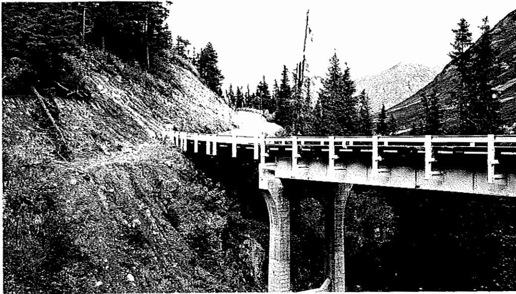
HJF-8. #900. Seward-Anchorage, Mile 54. View of old Pass Creek Bridge from upstream side. The approach spans on one end of bridge are on a 56-degree curve, and on the other end are on a 50-degree curve.
