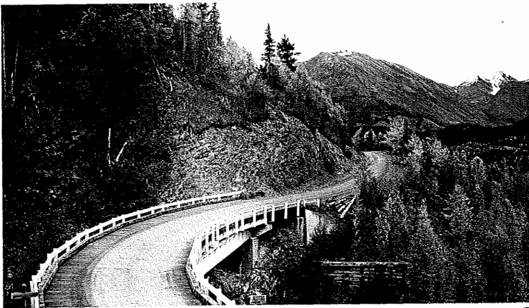
HJF-9. #903. Seward-Anchorage, Mile 58. View of Frenchy Creek Bridge from the south approach. Bridge is on a 45-degree curve. There are 325 degrees of curvature in less than 900 feet on these bridge approaches.
