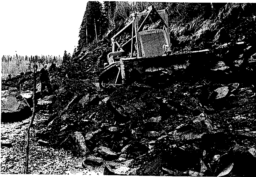
No. 663 - View of D-8 with dozer cleaning up cut at Sta. 148 after blast. View south May, 1950. Seward Forest Highway Project 3-A9.
