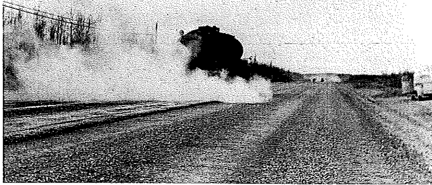
No. 656 - Distributor spreading MC-2 prime coat at 225 deg. F. View west from Sta. 295 in Ft. Richardson May 24, 1950. Glenn Highway Section A.
