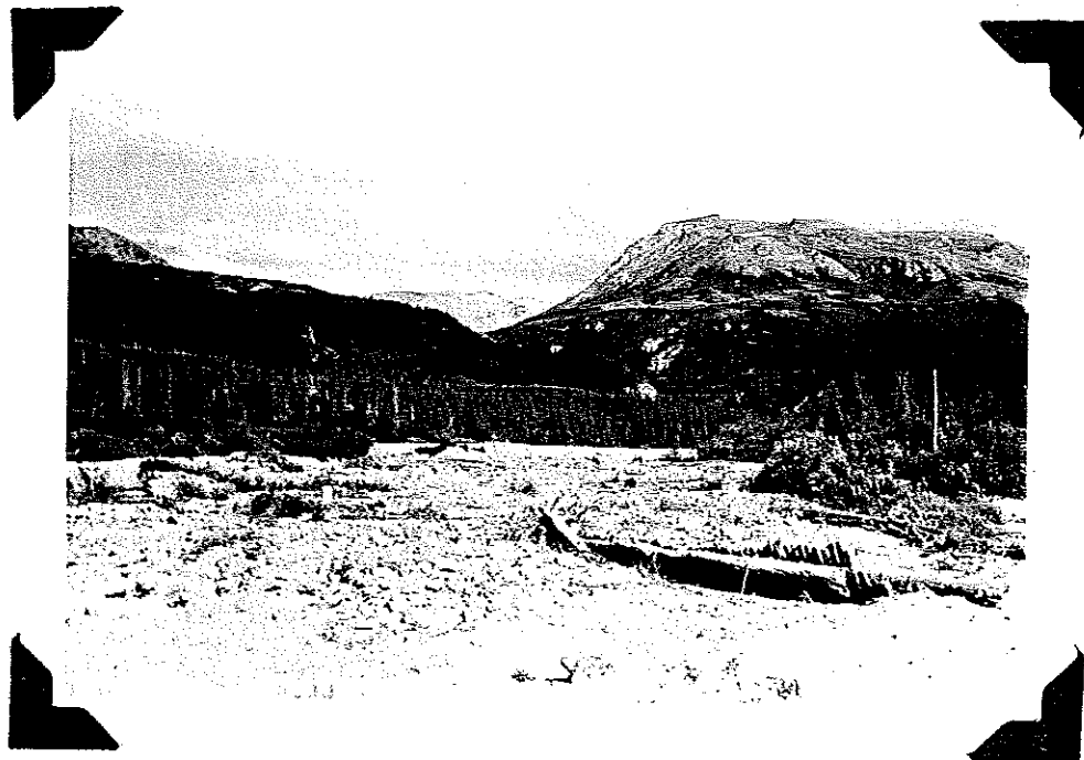
No. 742 - Richardson Highway Section C. (Big Delta - Rapids Survey) View of large wash below Rapids. Recommended line crosses wash at foot of hill in background where flow can be confined.
