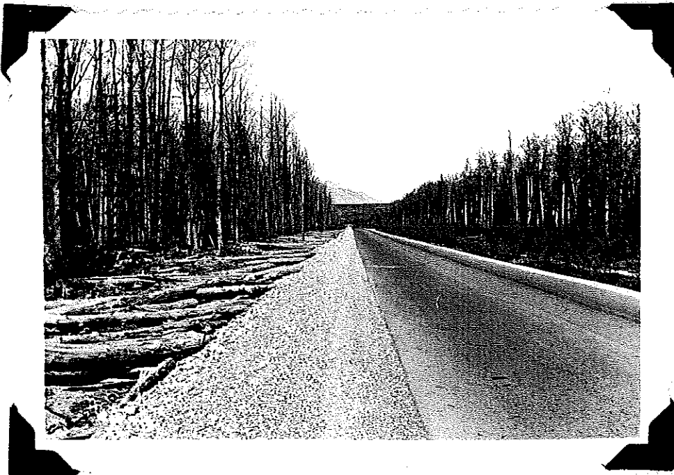
No. 672 - Glenn Highway. View of completed paving about 7 miles south of Palmer. Logs along fill have been decked to prevent erosion from Matanuska River flood waters.
