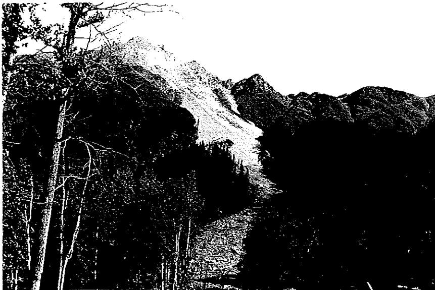
No. 731 - Glenn Highway Mile 38. View of large land slide that occurred in March 1950. The near end of the slide is about 200 ft. from the road. Upper part of slide is in constant motion. Rocks rolling down talus and the dust they stir up can be seen all the time. The grinding action of the slide can be heard constantly from the road.
