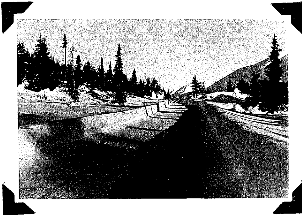
No. 500 - Winter scene at Mile 52 Seward-Hope road. The view is north and shows the typical road condition after the rotary plow has passed through. January, 1950.
