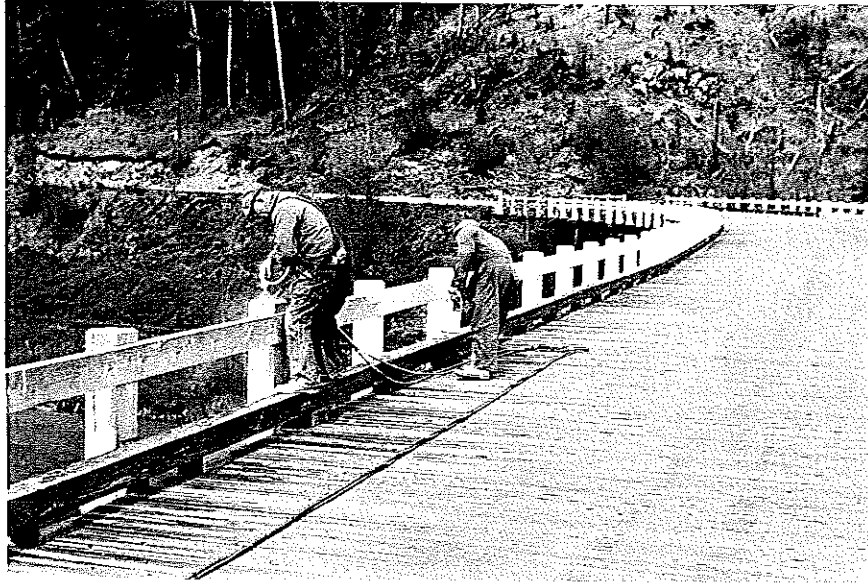
BHC-686 Seward Highway Maintenance. Shows maintenance employees painting Snow River Bridge at Mile 18.
