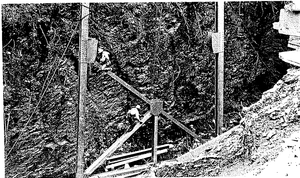
BVK 8-4 Turnagain Arm, Section C. Erecting steel bent on Dry Gulch bridge.
