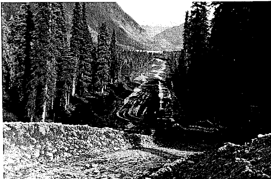
BGN 2-1 Kenai River Highway 5-B1. View of stripped muskeg section east from sta. 621+00.
