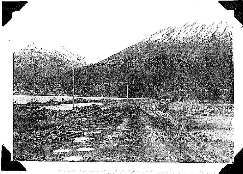
ENS 1-7 View of road between Seward and the airport. Shows driftwood deposited on road by extremely high tide accompanied by south wind on November 21. Tide washed over the road at this and several other points.
