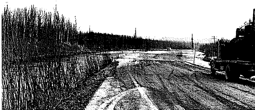
No. EHC 7-5 Salcha River overflowing road sta. 2111 to 2125 \frac{1}{2} on Richardson Highway project, sec. B. Looking east. May 15, 1949. Overflow caused by ice jam in river. Mile 325 from Valdez.
