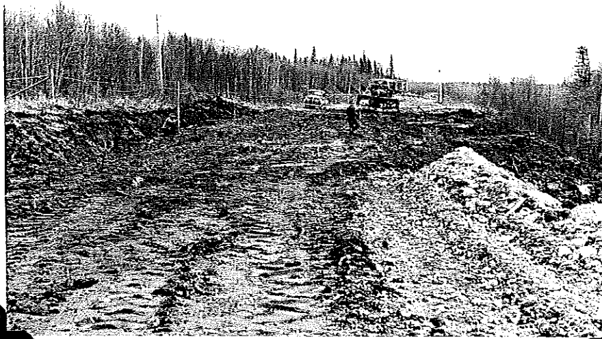
No. EHC 3-5. Subgrading unstable material at sta. 1642 on Glenn Highway project sec. A. Looking east April 28, 1949. Milepost 46 from Anchorage.
