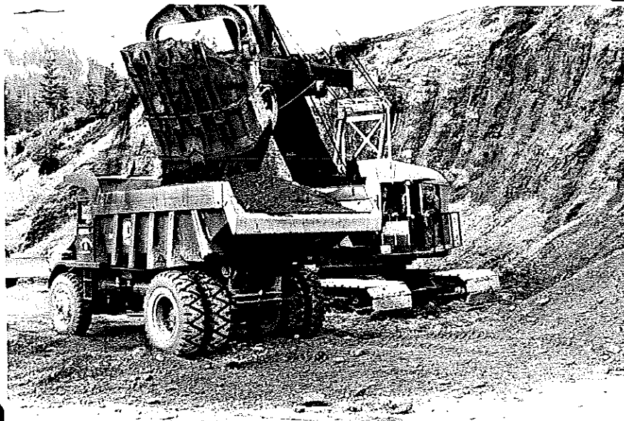
No. EHC 3-5 3 1/2 yd. shovel and 11 yd. truck working in borrow pit right of sta. 1304. Turnagain Arm project section F2. April 29, 1949
