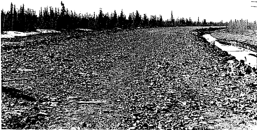
No. EHC 6-7 Looking northwest towards Fairbanks at rock borrow subbase completed at sta. 434 (8 miles from Fairbanks).
