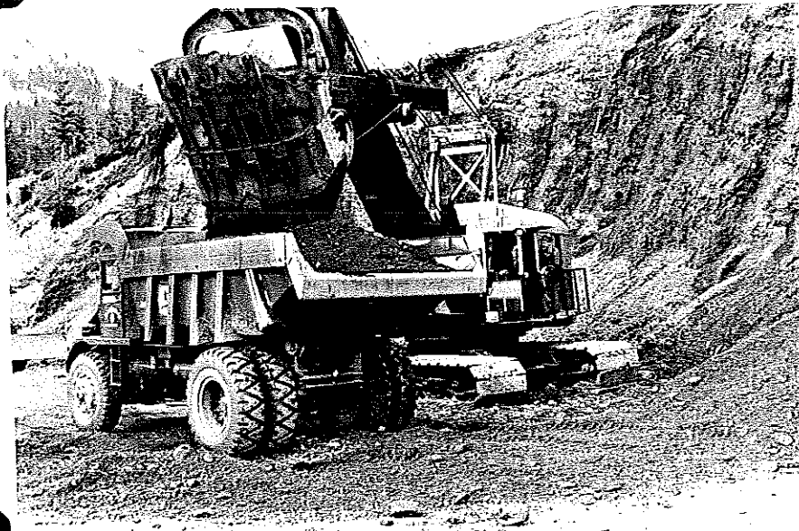
No. BHC 3-8 3\frac{1}{2} yd. shovel and 11 yd. truck working in borrow pit right of sta. 1304. Turnagain Arm project section F2. April 29, 1949
