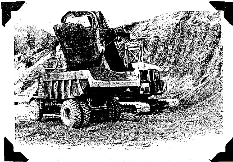
No. EHC 3-8 3\frac{1}{2} yd. shovel and 11 yd. truck working in borrow pit right of sta. 1304. Turnagain Arm project section F2. April 29, 1949
