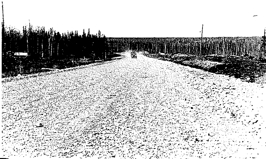
No. EHC 4-4. Looking north from sta. 1612/50 on Glenn Highway project sec. A at section subgraded and backfilled with select gravel borrow in 1948. May 2, 1949. Milepost 45 from Anchorage
