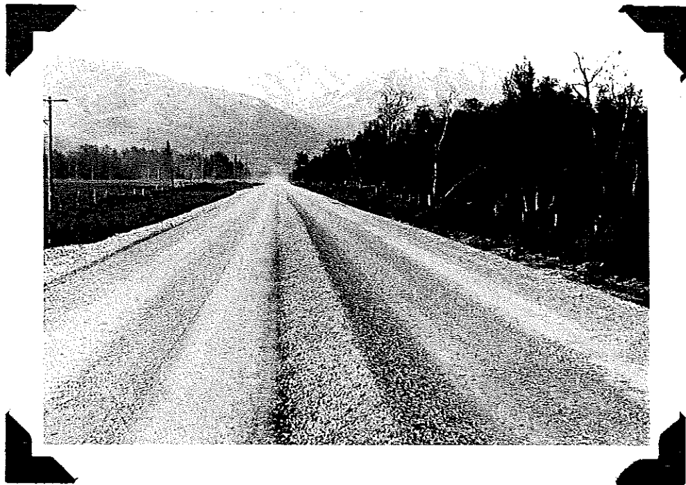
BMF 3-5 Glenn A. View south toward Anchorage from sta. 1950. This is the first tangent south of Palmer. Shows base course in windrow partly processed.
