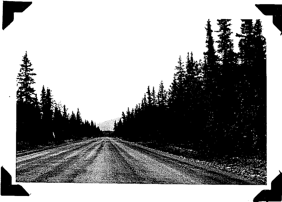
BMF 3-6 Glenn A. View north (toward Palmer) from Sta. 1575 (Mile 40.6). Shows compacted base course.
