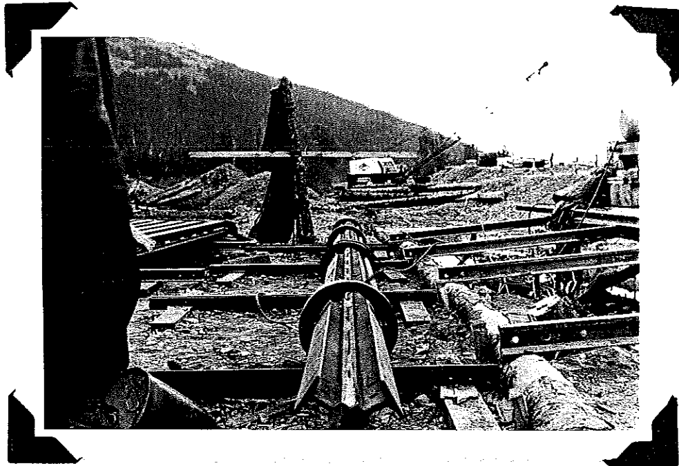
BMF 4-1 Shows device used to hold rails during welding. Turnagain Arm F3 Bridges, July, 1949.
