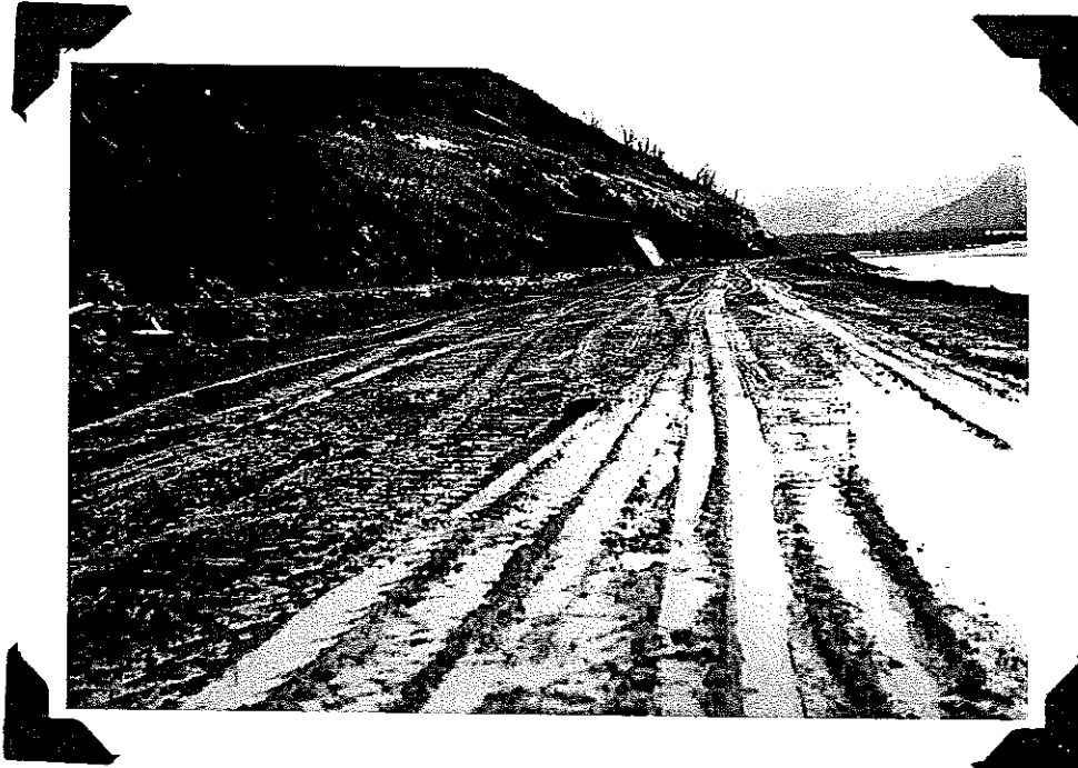
RWS 4-4 Rough grading completed for combined highway and railroad fill. Looking back and east from sta. 1405. Present railroad to be moved to outside of new fill. Turnagain Arm on right. November, 1949.
