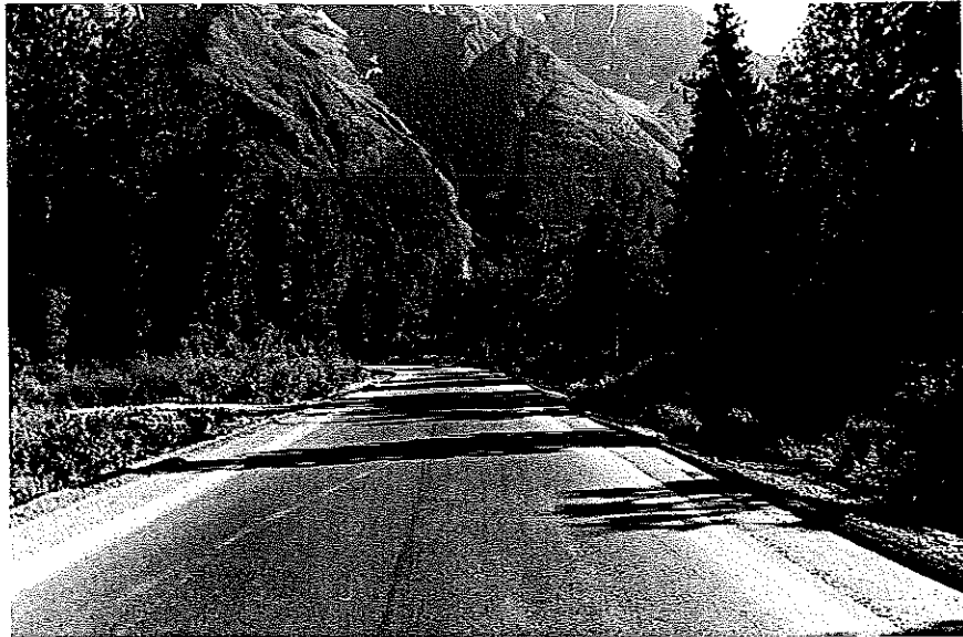
B.M.F. 5-2 Glenn Highway, Section A. August 10, 1949 Back from 1530. Shows completed plant mix. No seal or chips on.
