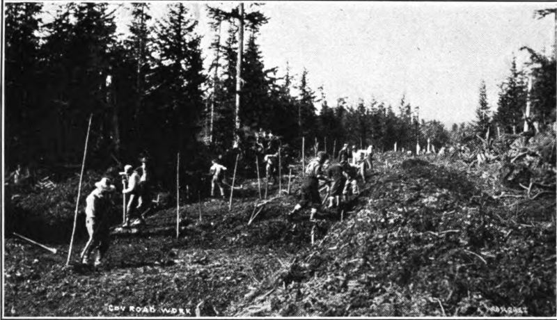
STRIPPING ROADBED, AUK BAY EXTENSION.
