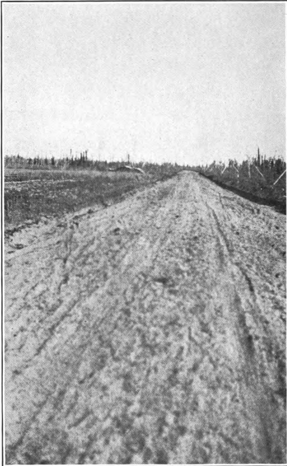
MILE POST 367½, ROUTE 4K, VALDEZ-FAIRBANKS ROAD.
