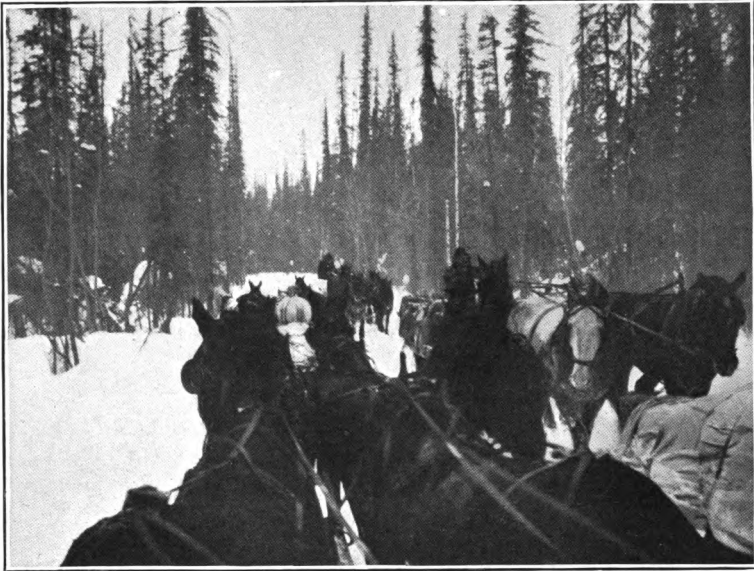
SLED ROAD, FAIRBANKS TO WASHBURN.
