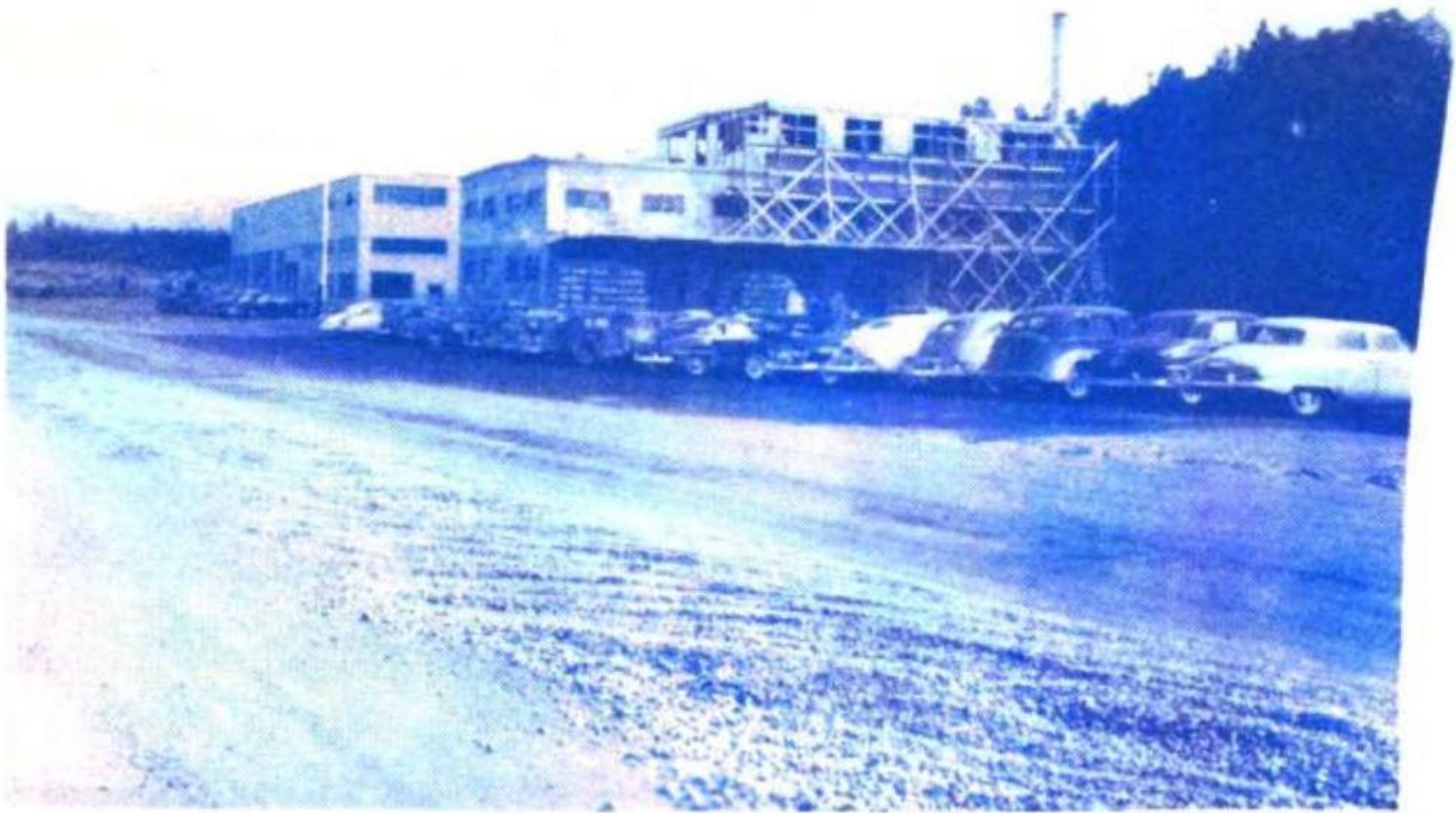
Penthouse addition for the Anchorage District Office at the Anchorage Depot. Construction completed January 1951.
