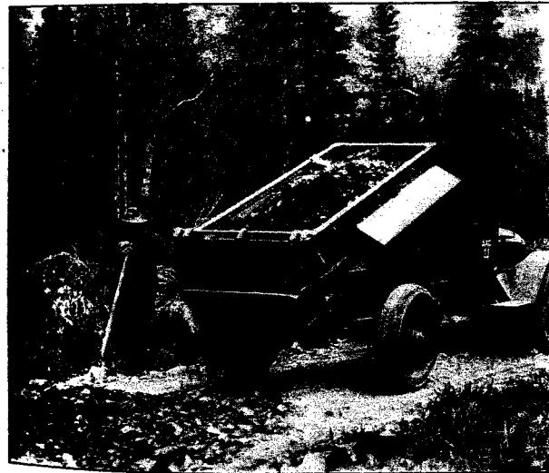
PLACING SURFACING NEAR CHITINA, RICHARDSON ROAD.
