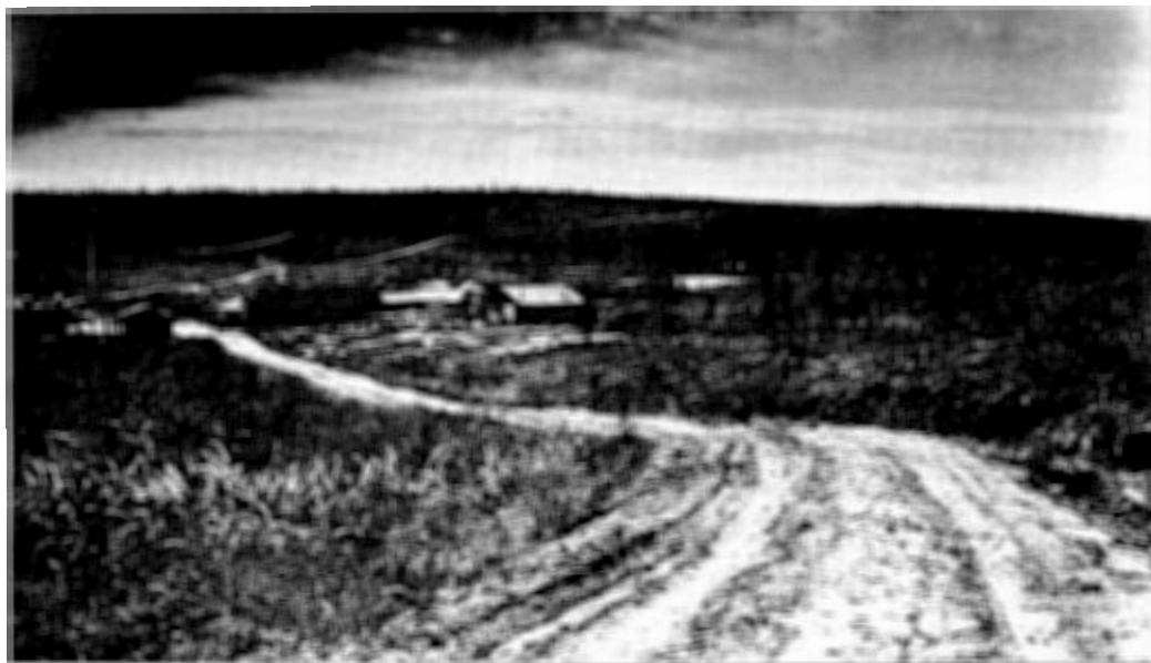
Until eligible for funding under the FAHA, Alaska had little control over development of its road system. (Huddleston Collection, APRD)
