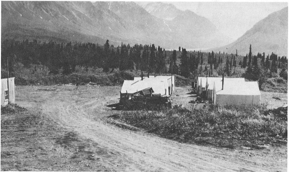
Construction camp at mile 68, Glenn Highway, 1944. AMHA.
