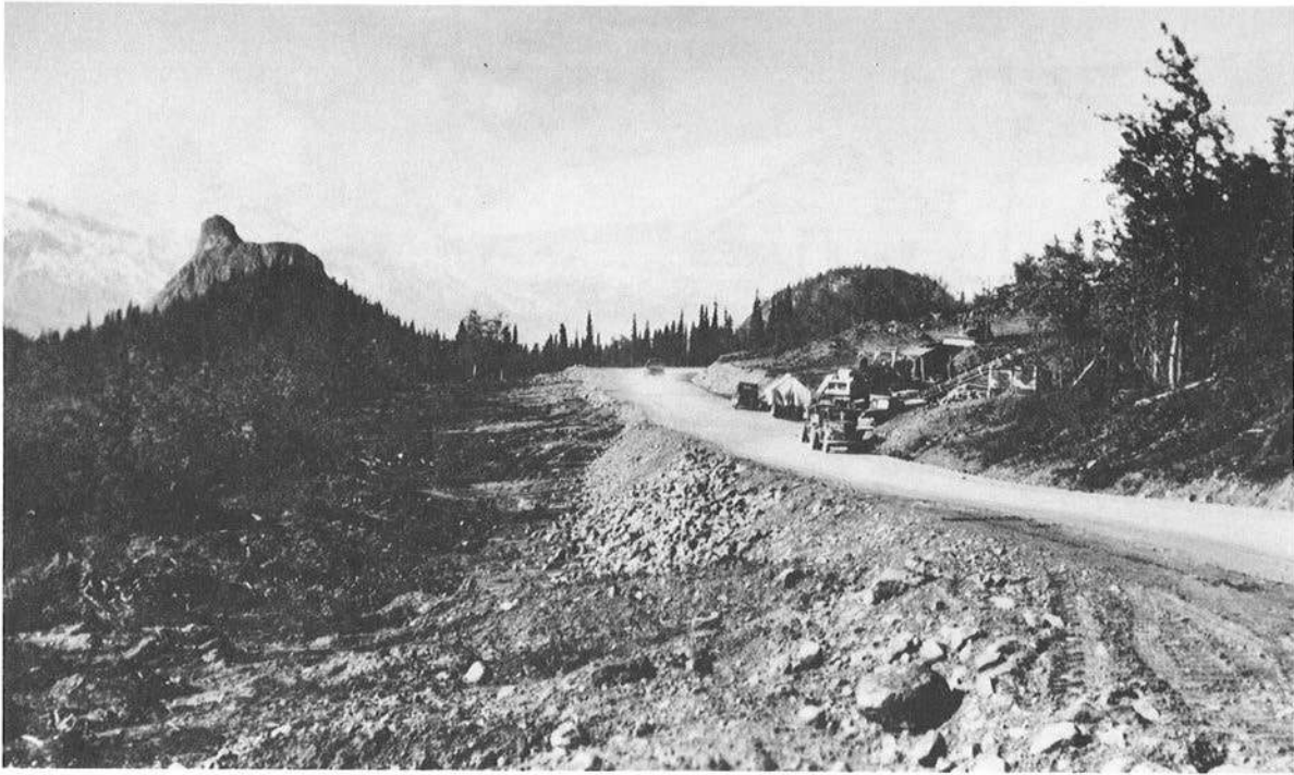
Glenn Highway construction, 1944. AMHA.
