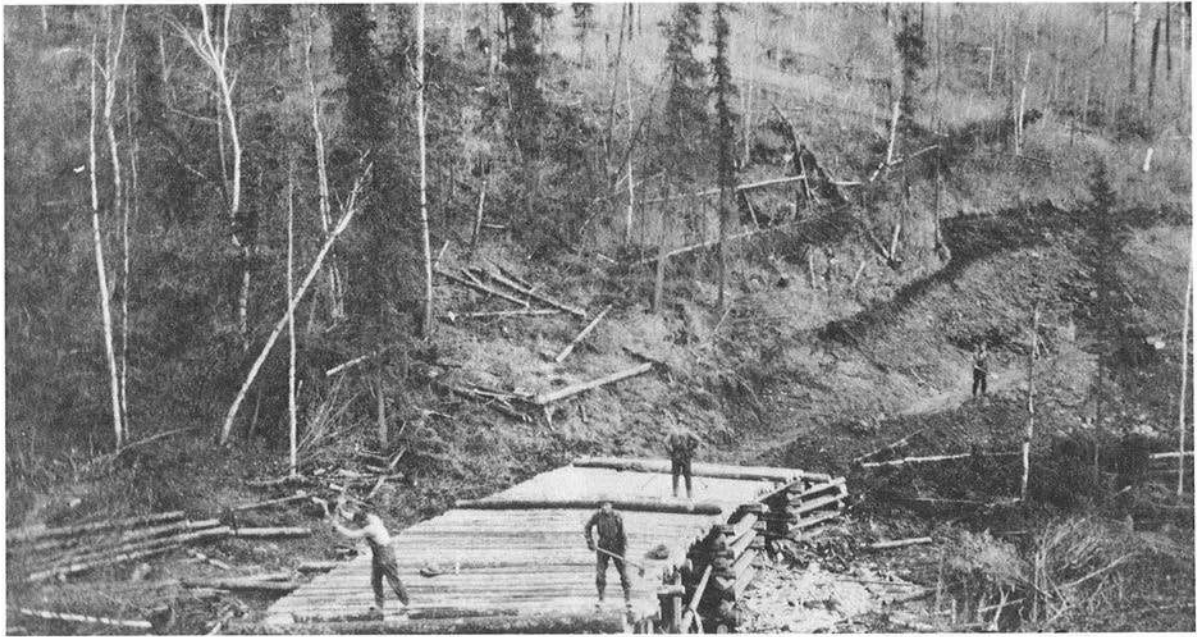
Bridge construction on the Richardson trail, about 1913. John Zug Collection, UAF.
