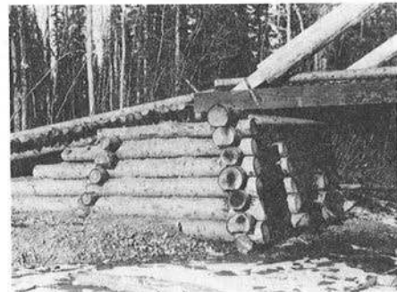
Bridge construction detail, about 1913. John Zug Collection, UAF.
