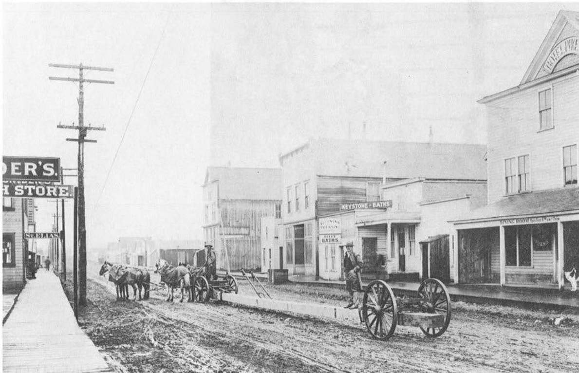
Bridge timber for Alaska Road Commission, cut by the Copper River Lumber Co., Valdez, about 1912. John Zug Collection, UAF.
