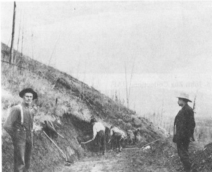
Work crew digging embankment, Richardson trail, about 1913. John Zug Collection, UAF.
