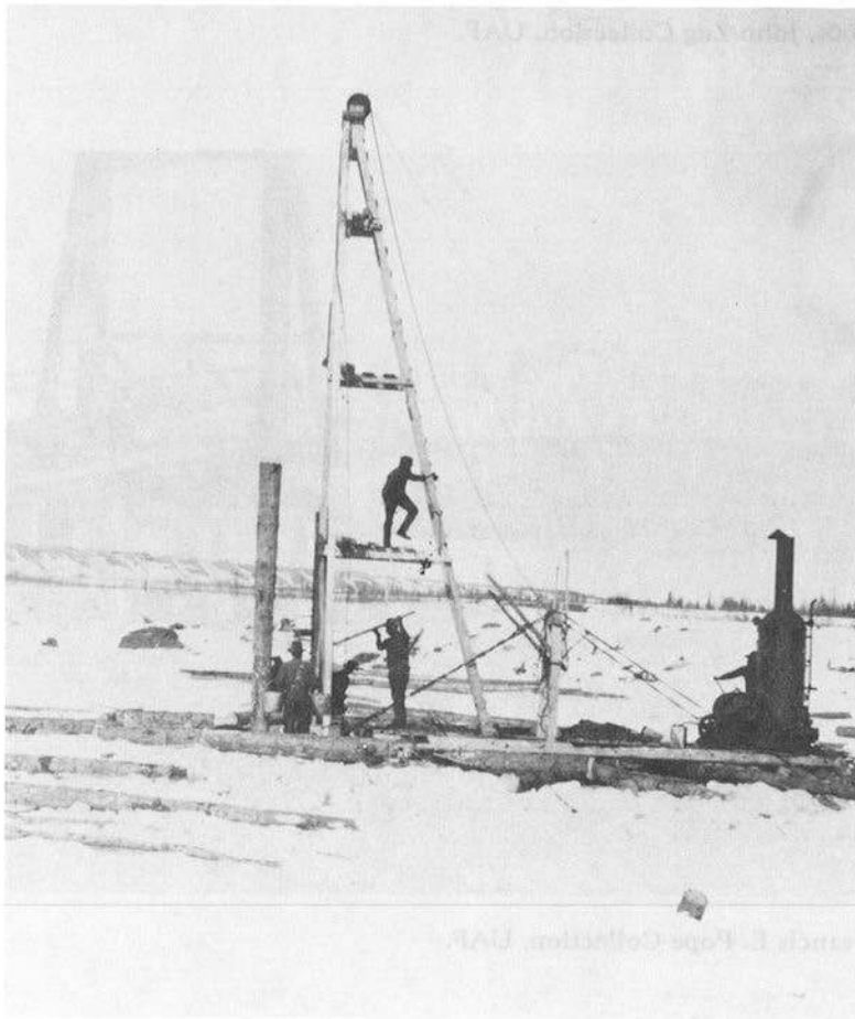
Pile driver in operation on Tazlina River bridge, 1906. Francis E. Pope Collection, UAF.
