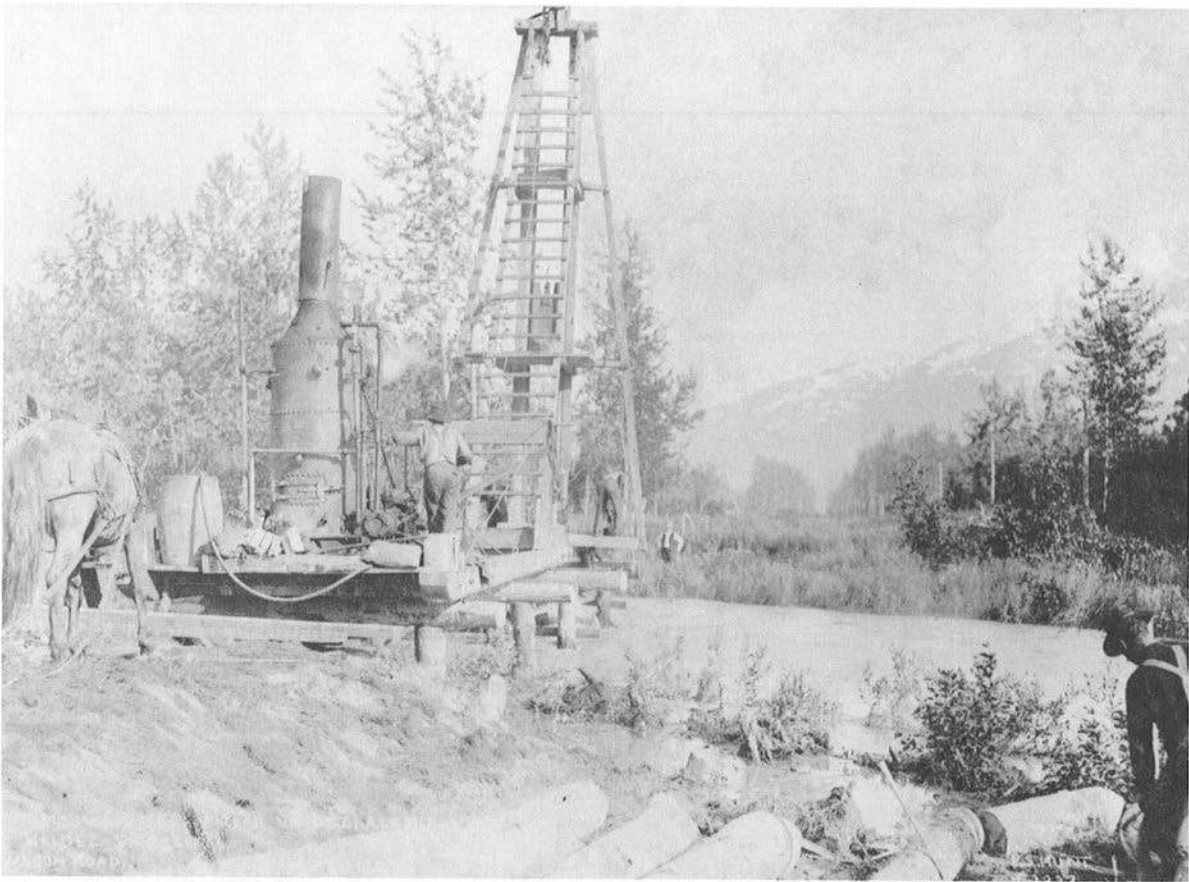
Boiler and pile driver in operation on bridge construction near Valdez, about 1910. John Zug Collection, UAF.
