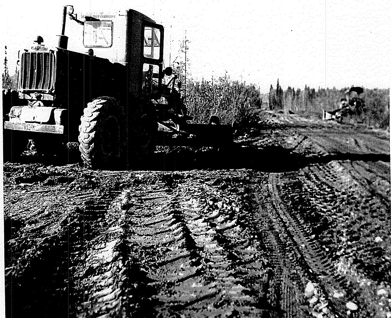
FIG. 3-2 Chena Hot Springs road - re-building fill in low marshy area in previously constructed section.
