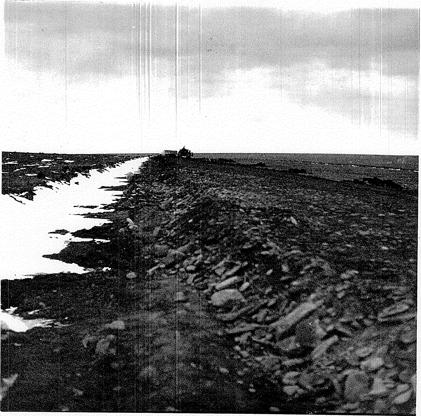
Fig. 33-P US 97 - Nons. Typical fill section placed by contractor.
