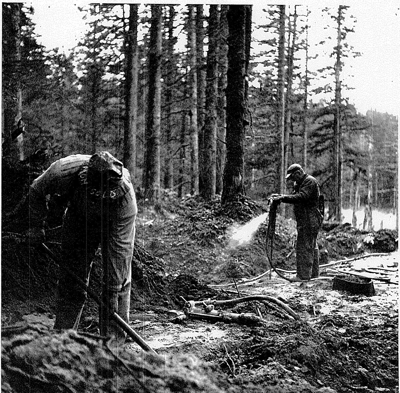
**Fig. 22-E** Kodak - The men drilling and shooting at quarry.
