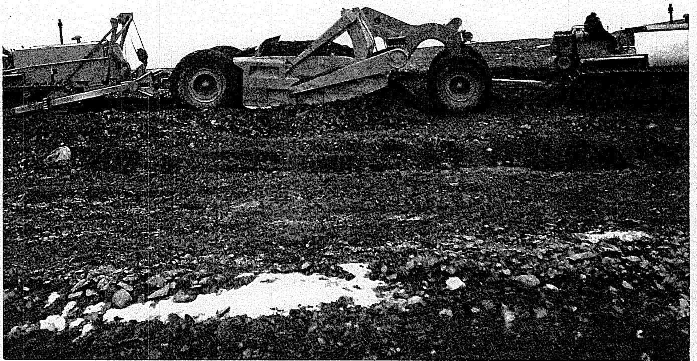
Fig. 32-a US 97 Zone; cut and can with push cut working borrow pit.
