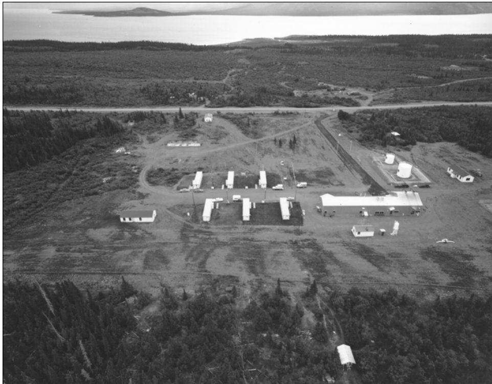
Figure 34. Destruction Bay Pump Station. NARA.
