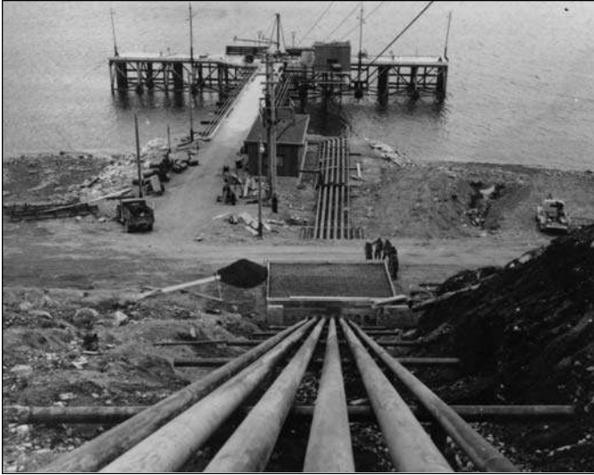
Figure 16. Pipes leading from Haines dock to manifold building. NARA.
