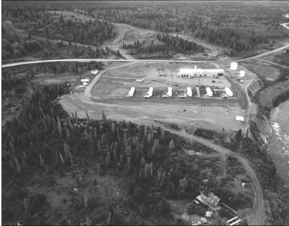
Figure 33. Blanchard River Pump Station. NARA.
