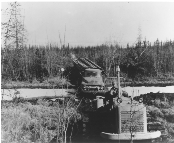
Figure 4. Push and Pull assistance was necessary to bring piping to the places needed in tundra swamp crossing. NARA.
