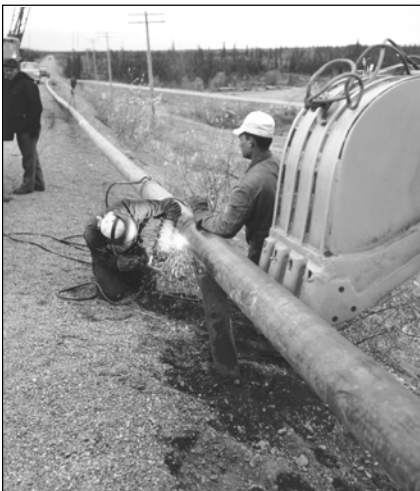
Figure 7. Pipe welding. NARA, DA 573 #373.
