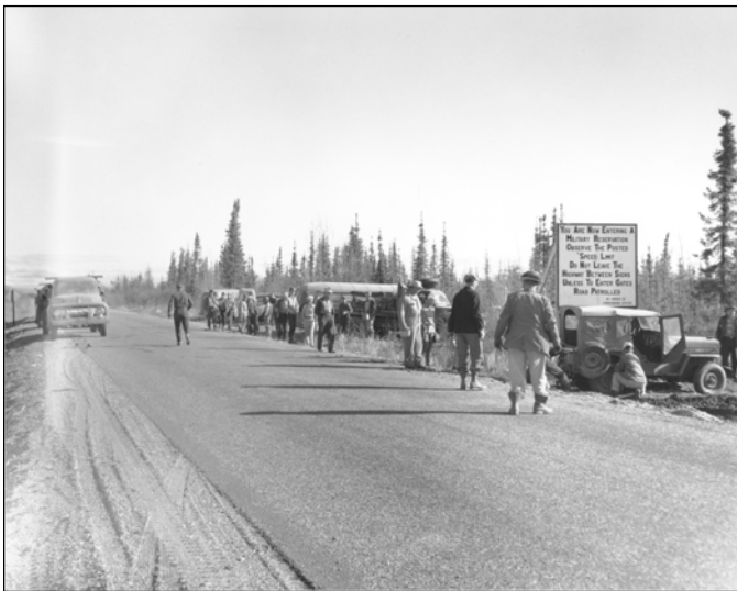
Figure 12. 1954, Mile 28. Workers assemble on highway.
