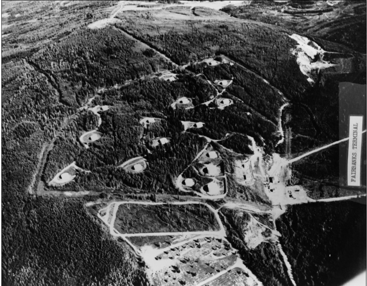
Figure 29. Aerial view of Fairbanks Terminal. University of Alaska Anchorage: Consortium Library Manuscripts & Archives Dept. U.S. Army Haines Fairbanks-Pipeline Records 1954–1958.
