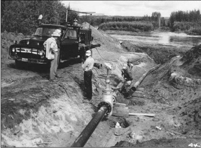
Figure 5. Laying pipe for underwater crossing. NARA, A4-3826.
