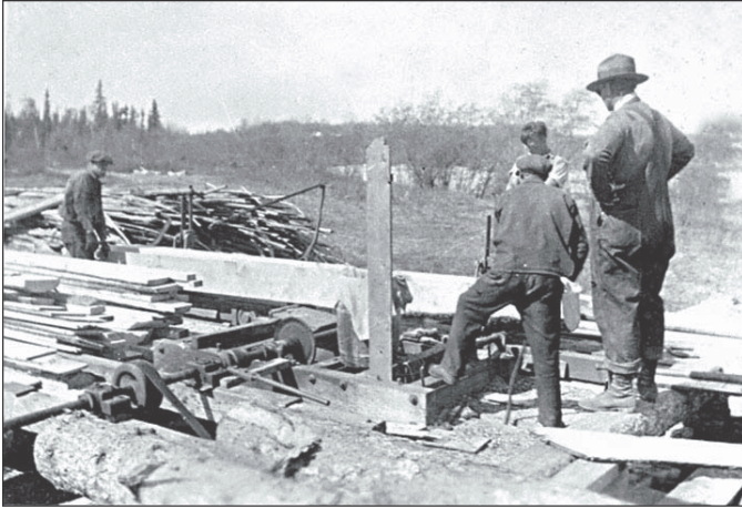
Figure 25. Planking saw in operation. Chester Spencer is standing at right. Courtesy of Ted Spencer.
