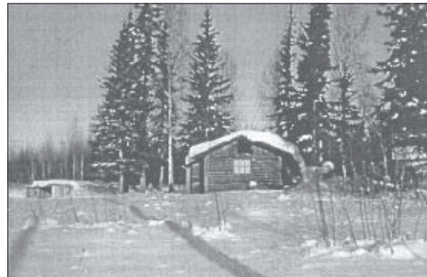
Figure 35. Nodackers' cabin, south elevation ca. 1953. Corps of Engineers photo.
