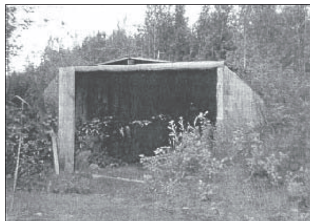
Figure 37. Nodackers' dugout garage ca. 1953. Corps of Engineers photo.
