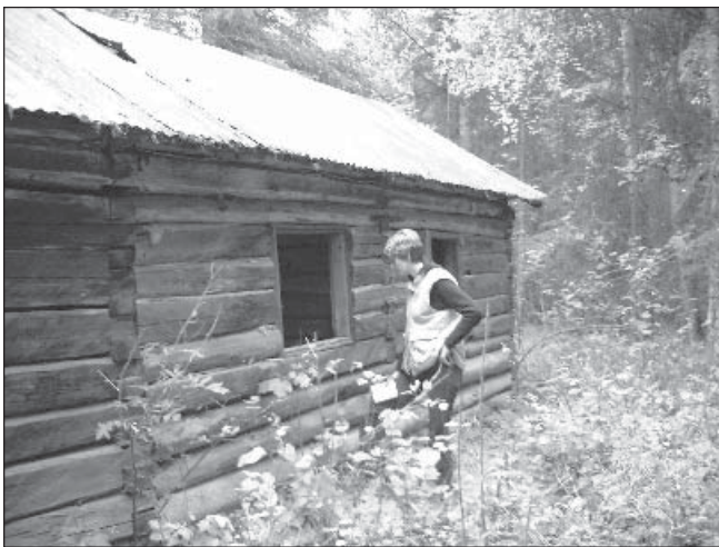
Figure 27. East view of Mannick cabin. From collection of USARAK.
