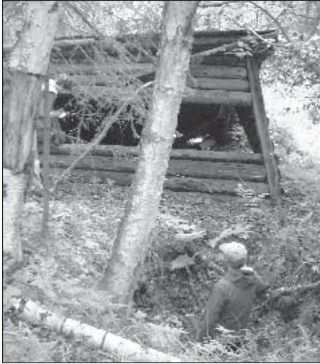
Figure 26. Front view of Meier cabin. Bill Quirk standing in storage pit to right. From collection of USARAK.
