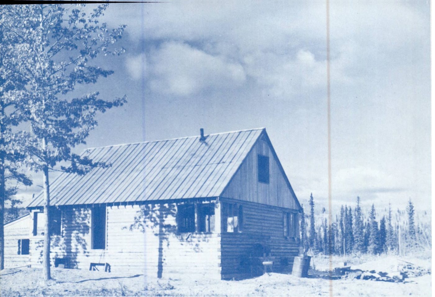
THIS MODERN, well-constructed house near Fairbanks was built of native "3-squared" timber, insulated with sawdust, and roofed with aluminum. Construction costs are extremely high.
