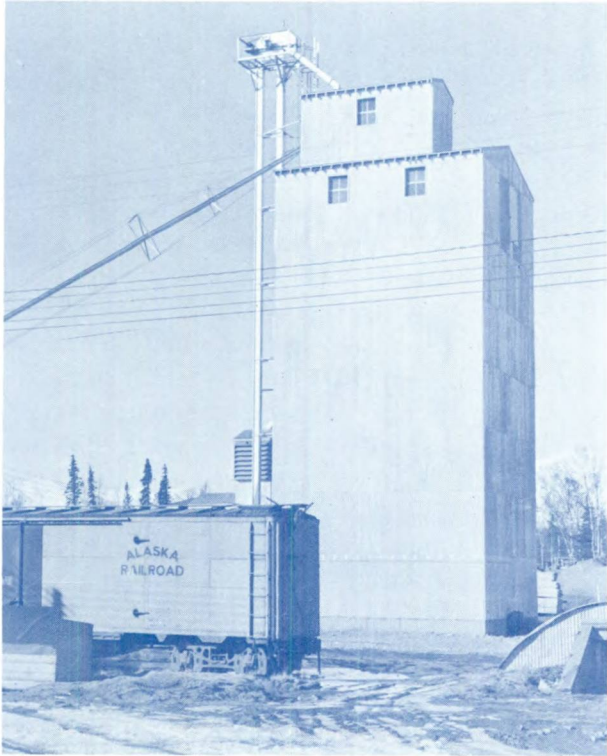
THIS COMMERCIAL GRAIN STORAGE and drier in Palmer, northeast of Anchorage, is the only one in Alaska.
